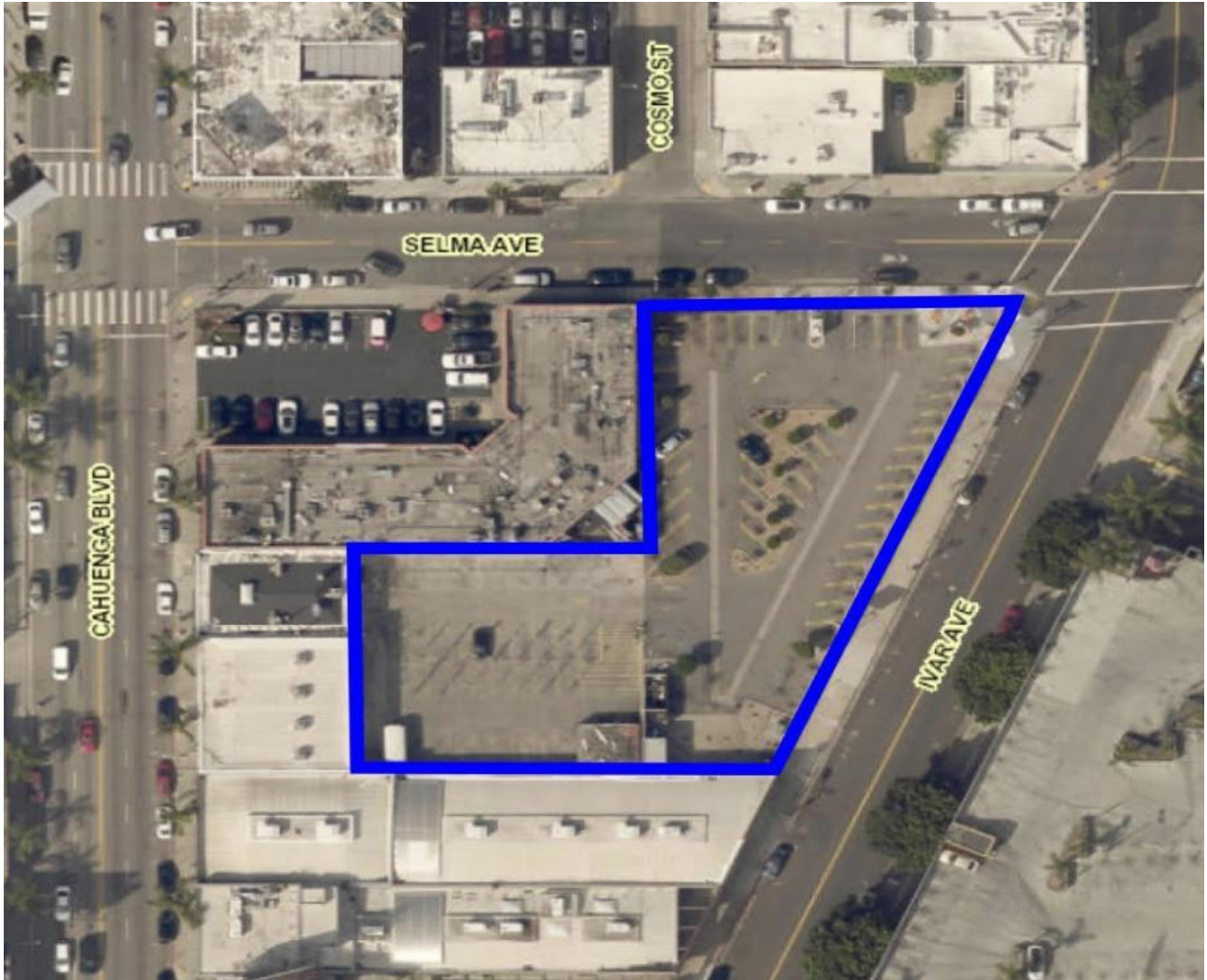
Aerial image of subject property 6350 W. Selma Avenue, Los Angeles Image Source: Zimas
