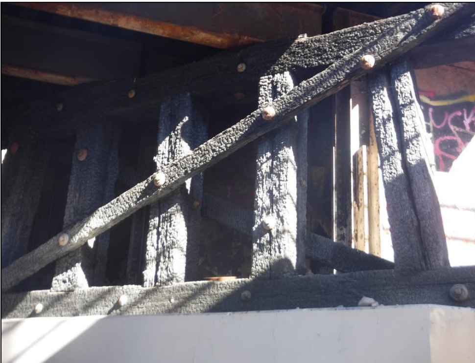
Photo 3: Typical split columns (photo of pony bent at Pier 6).
