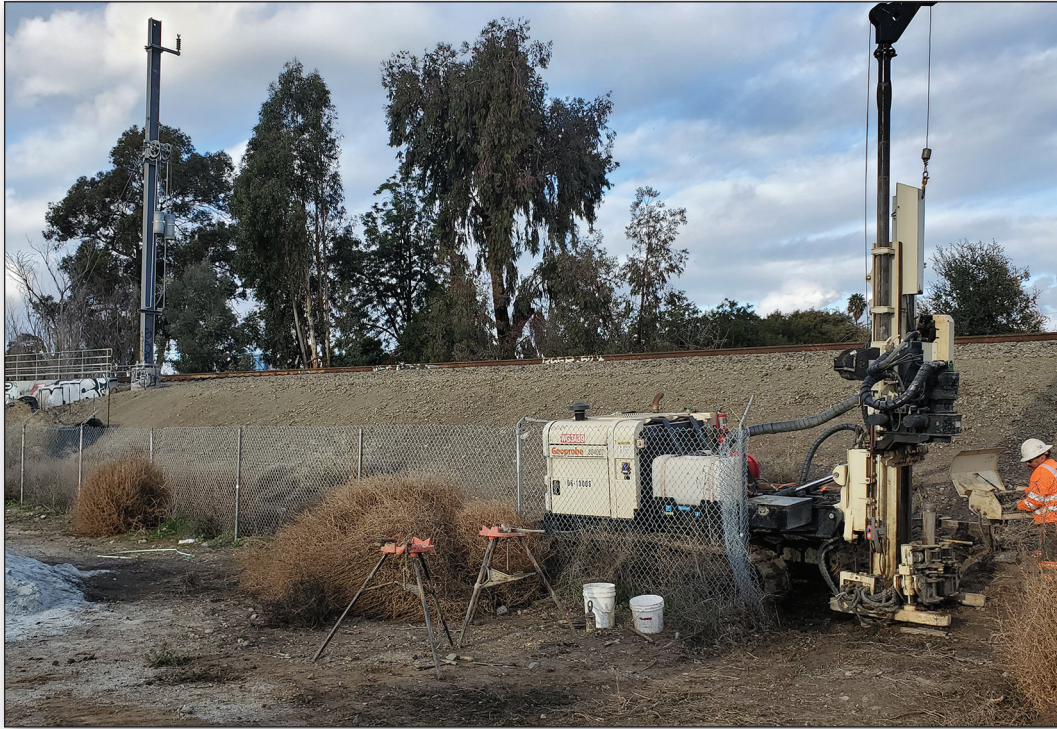
Drilling Core 2, view to the north.
