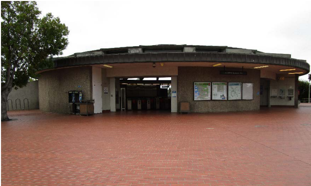
Figure 3 North Berkeley BART Station Building, South Elevation, Facing North
