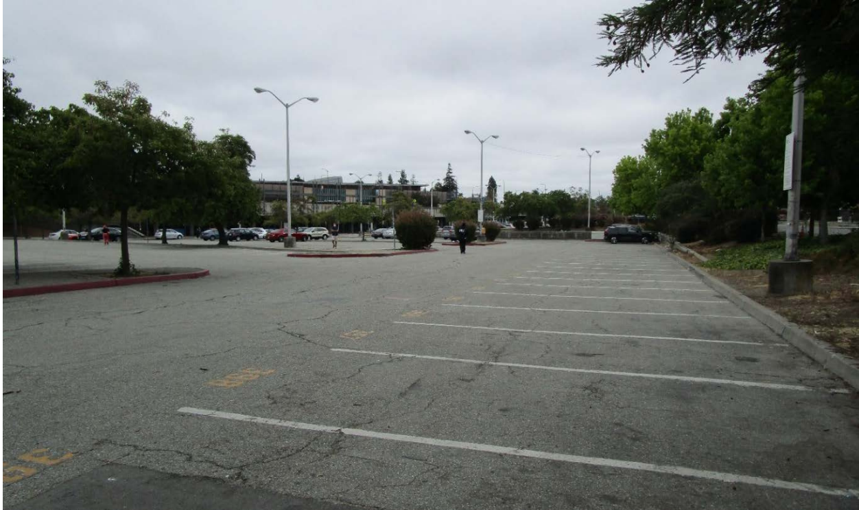
Figure 20 Ashby BART Station Parking Lot near Martin Luther King, Jr. Way, Facing Southeast
