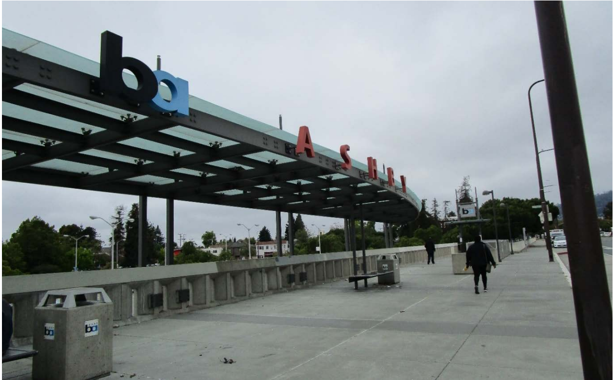
Figure 16 Ashby BART Station, Street-Level Deck along West Side of Adeline Street, Featuring Non-Original Canopy and Signage, Facing Northwest
