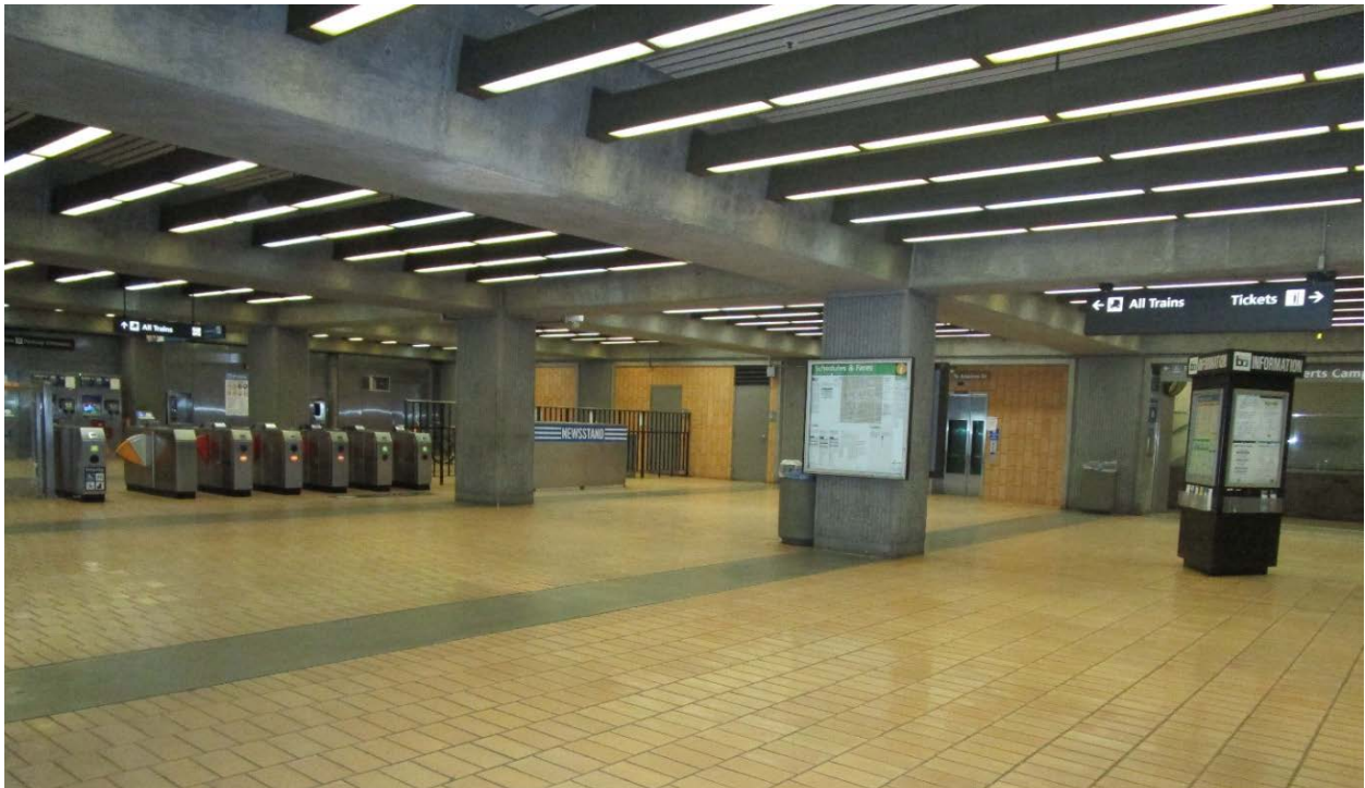
Figure 17 Interior View of Entry Area of the Ashby BART Station Concourse Level
