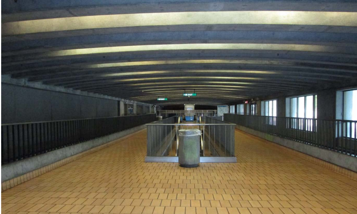
Figure 18 Interior View of Paid Area of the Ashby BART Station Concourse Level
