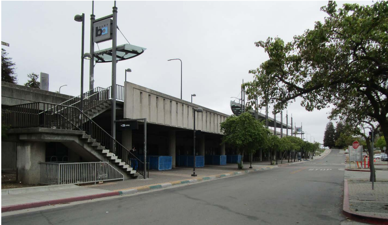
Figure 4 Ashby BART Station, West Elevation, Camera Facing Southeast
