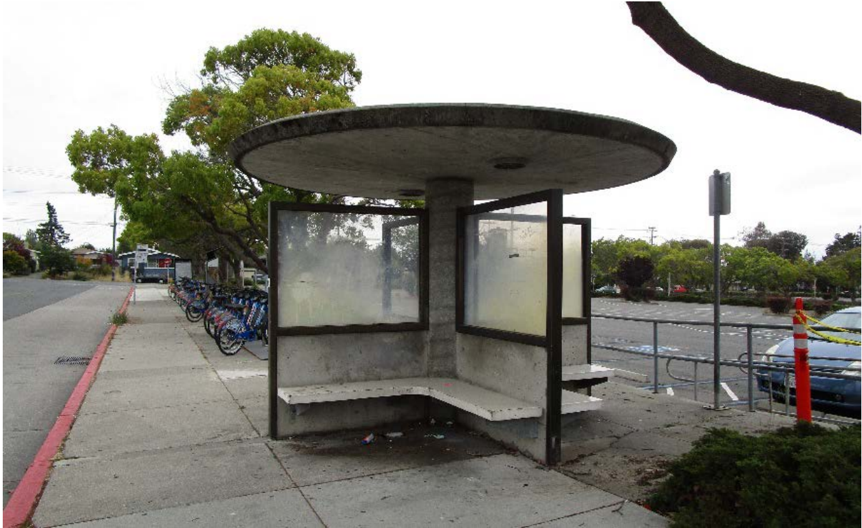
Figure 14 North Berkeley BART Station Bus Shelter, Facing Southwest
