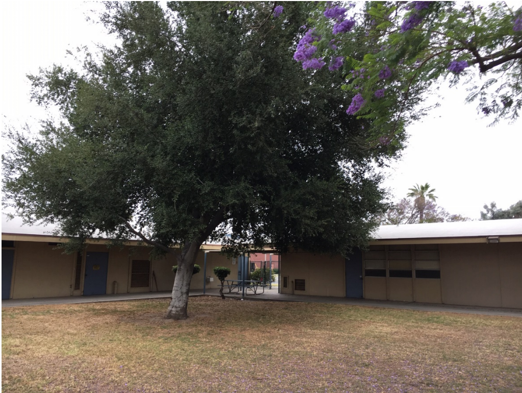
Photograph 4: View of the existing buildings and landscaped vegetation.
