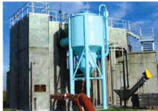
Hydro-Grit™ Vortex Grit Separation System
