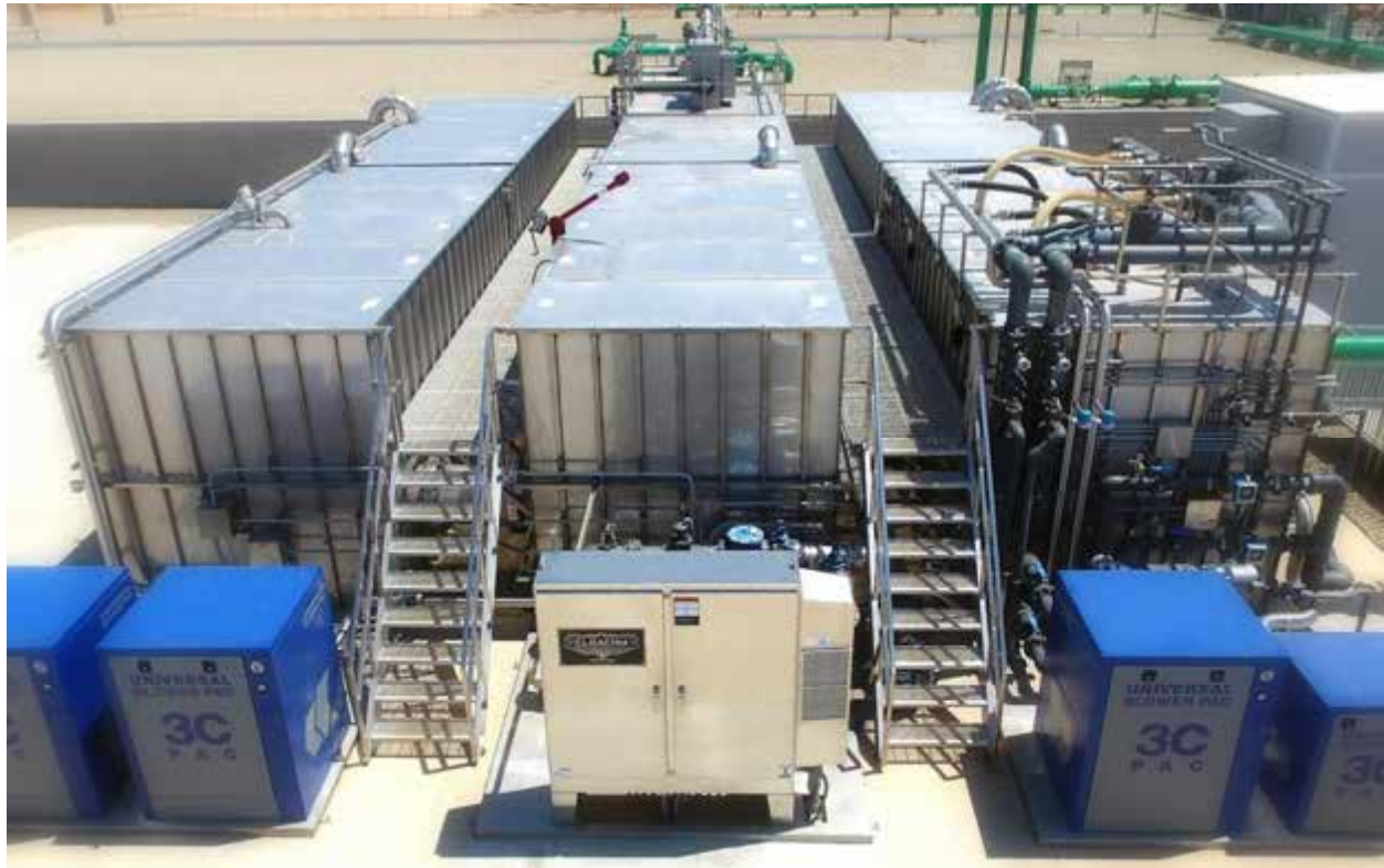
Figure 4-3: Example of Pre-Engineered, Packaged MBR Treatment Plant (Cloacina, 2019)
