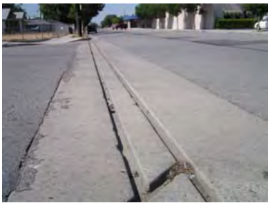
Bicycle unfriendly slot drain
