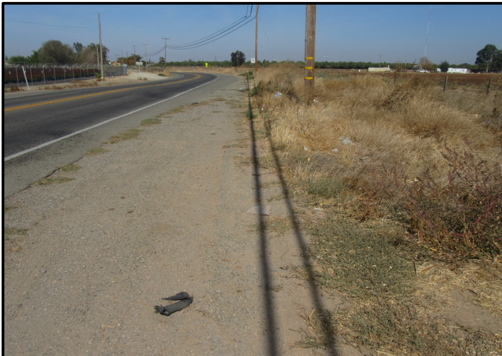
Location of the pipeline alignment along the east edge of Hickman Road, looking north from near Delaware Road; 10/15/19. The alignment will be placed in the east lane within the existing pavement.
