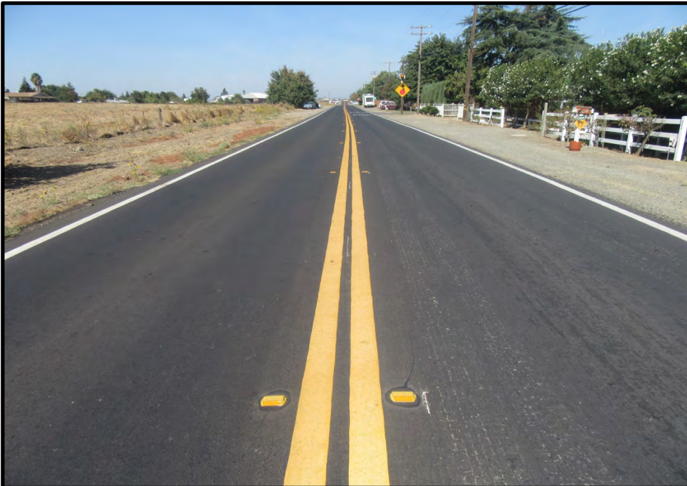
Center of Montpelier Road, looking northwest from approximately 300 feet south of the intersection of Fourth Street and Montpelier Road; 10/15/19. The pipeline alignment will be placed in the pavement on both sides of the road.
