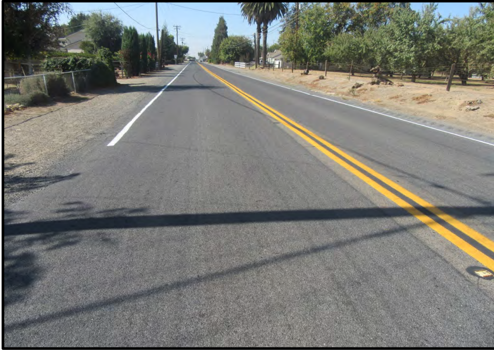
Lake Road, looking west from the intersection of Lake Road and I Street; 10/15/19. The pipeline will be placed on both sides of the road, along the pavement and road shoulder.
