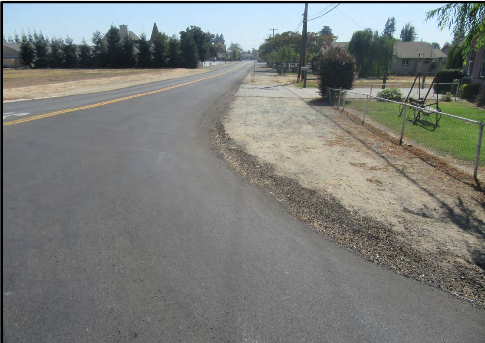
Road shoulder along the west edge of I Street, looking southeast from the intersection of I Street and Lake Road; 10/15/19. The pipeline will be placed along the west edge of the road, which is primarily graveled.
