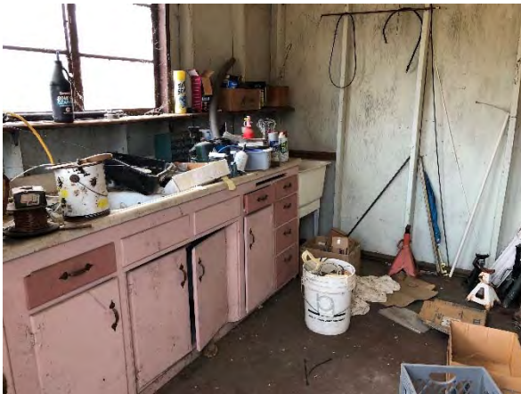
Photo #15 View of the interior of the storage shed, facing east.
