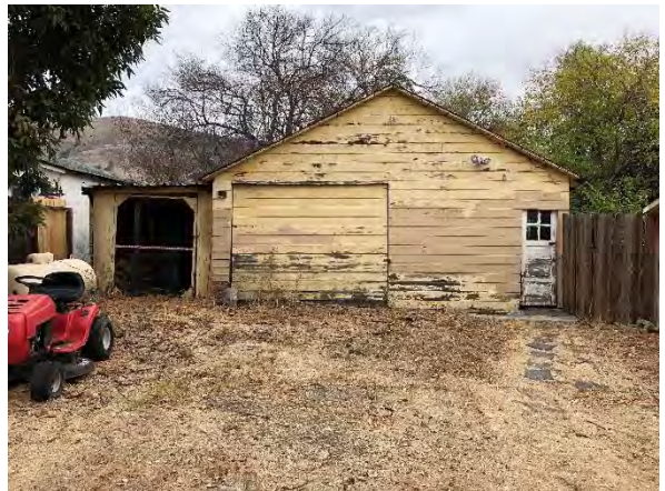
Photo #4 View of the front of the garage, facing northeast.
