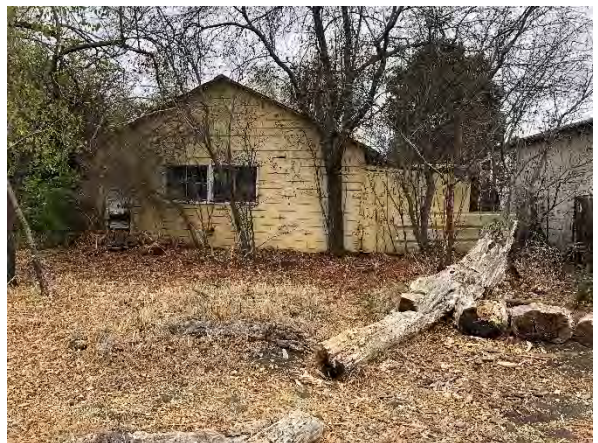
Photo #6 View of the rear of the garage, facing southwest.
