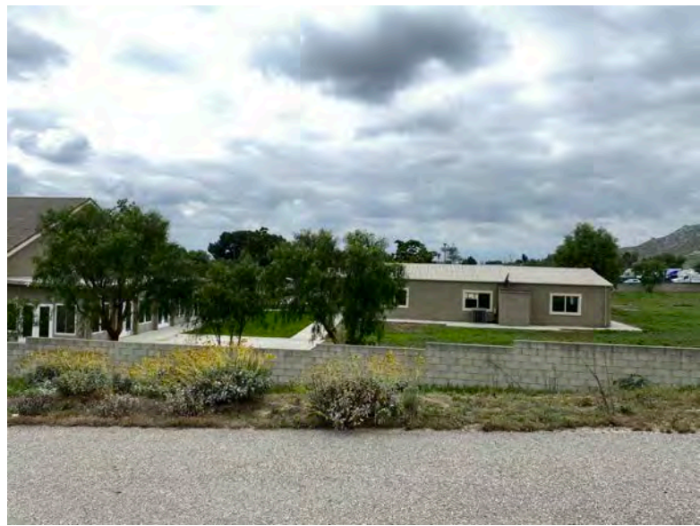
Side and Rear Yard of Church
