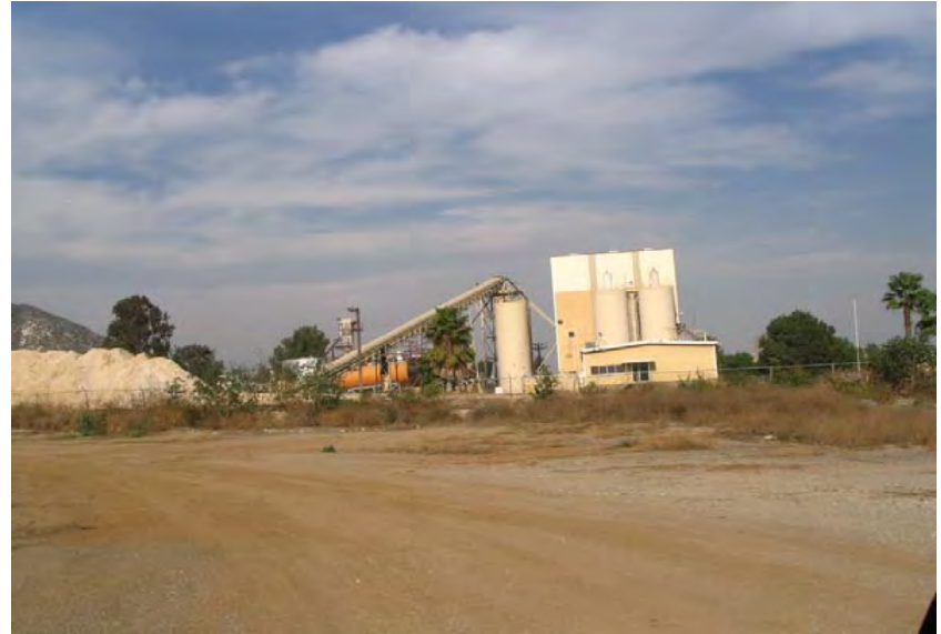
10. View of sand milling plant adjacent to north of northern parcel.
