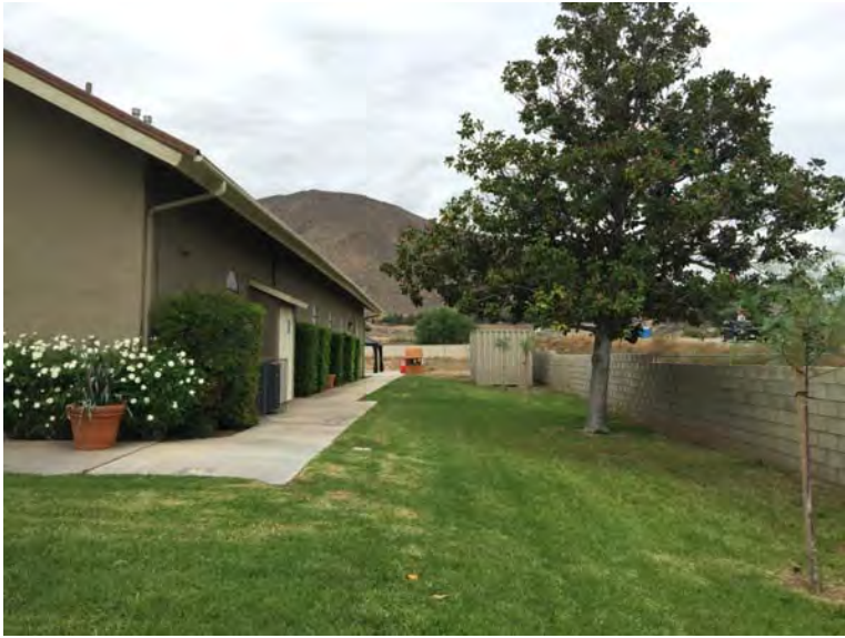
Side Yard With Storage Container Visible
