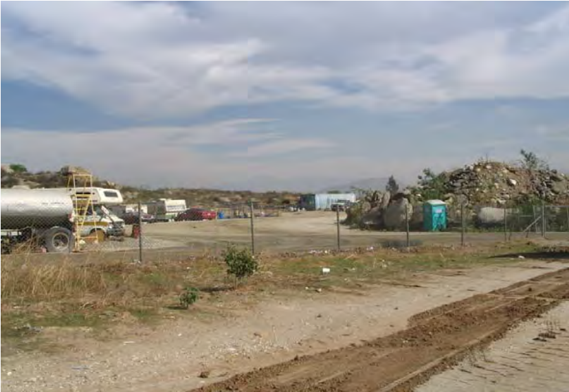
5. Southern portion of northern parcel with trailer and miscellaneous storage. Tanker truck at left foreground is water for dust control.
