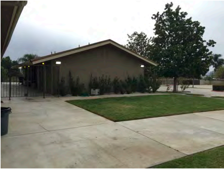
Second Accessory Structure
