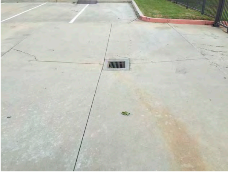
Stormwater Drop Structure
