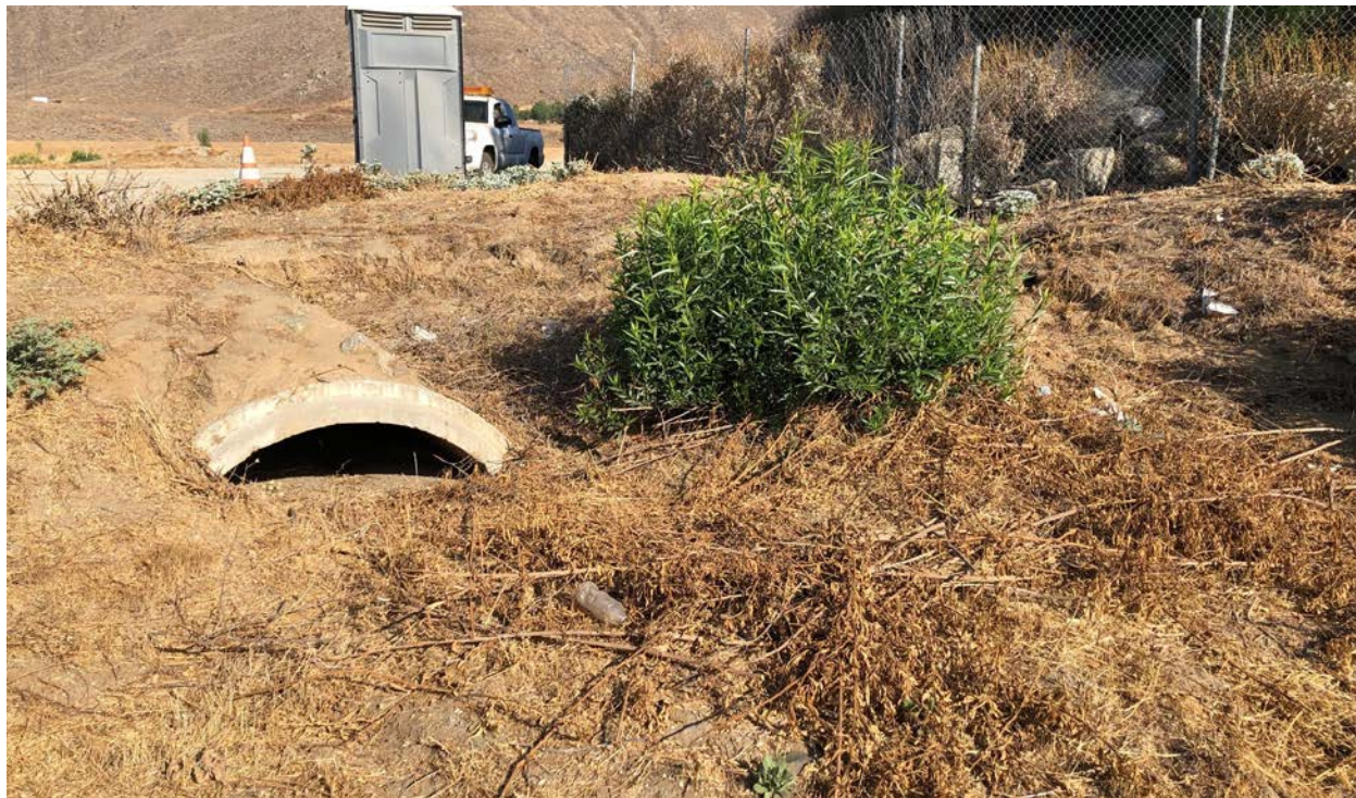
Photograph 3: Downstream view of West Riverside Canal at mostly buried culvert at 26 th Street. Note dense upland vegetation within abandoned canal.
