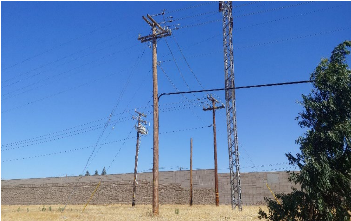
Utility Poles on the project site
