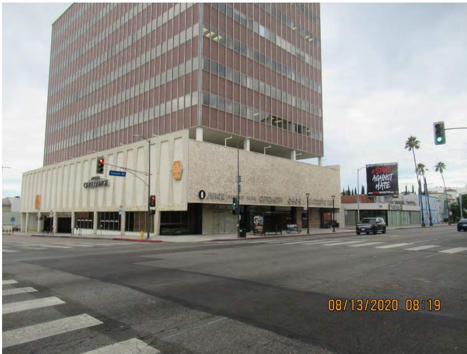
4. Adjacent property to the west across Wilcox Avenue (looking from across Sunset Boulevard to the south).
