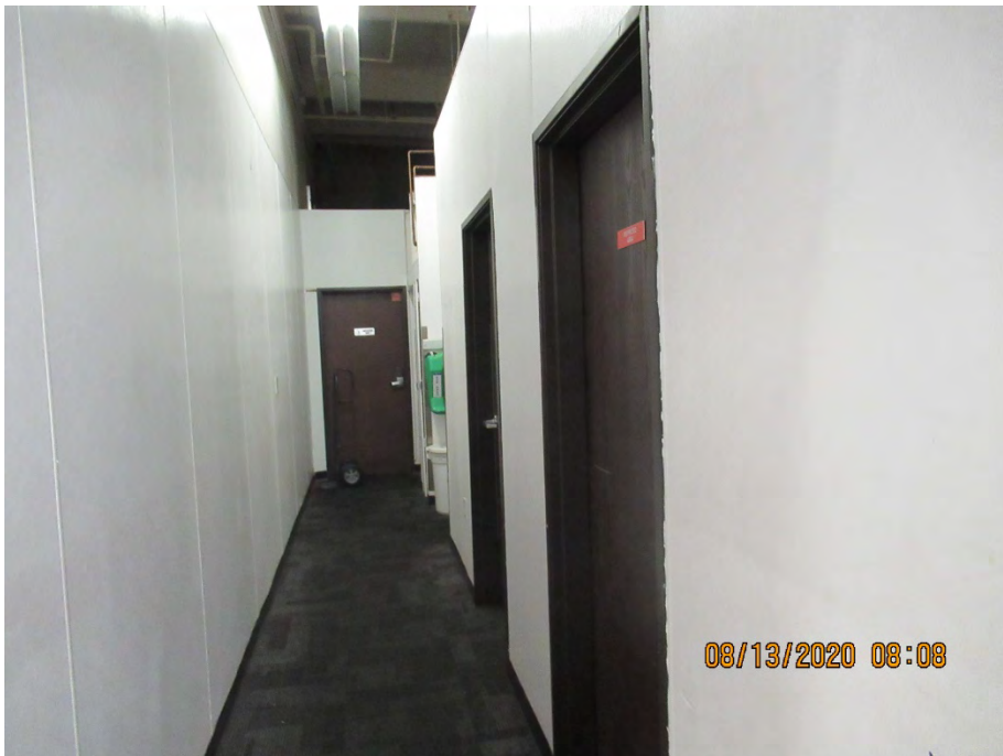
12. Restrooms and rear office area.
