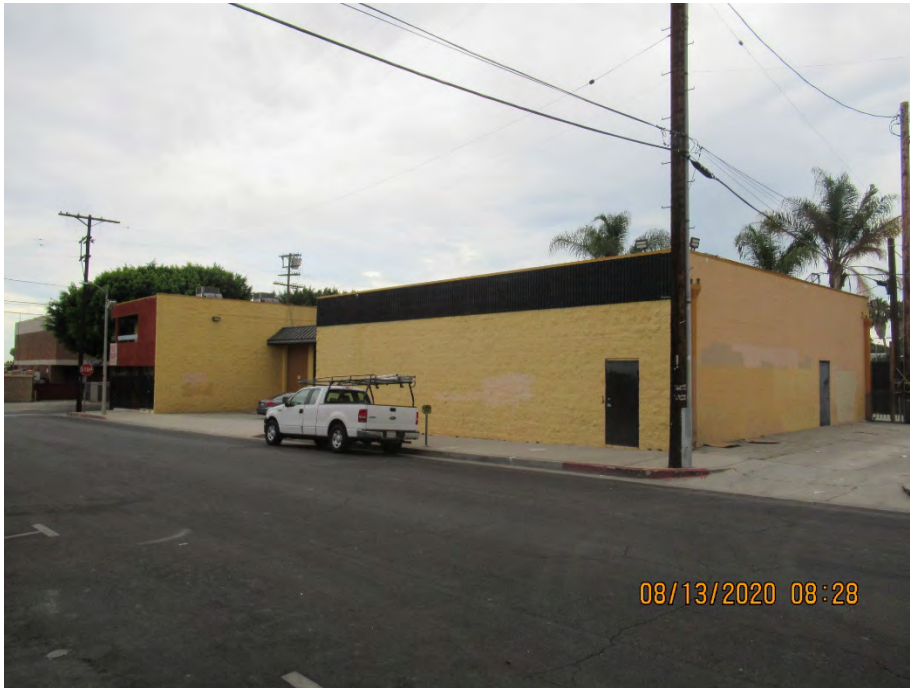
3. Additional view of adjacent property to the south of the subject site following an alleyway.
