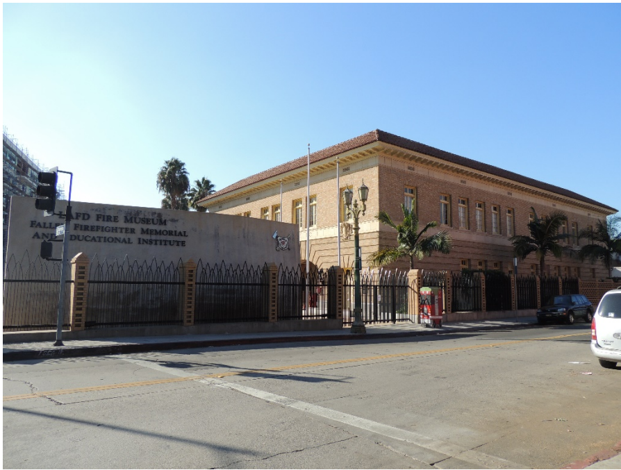
Fire Station No. 27, view facing southwest.
