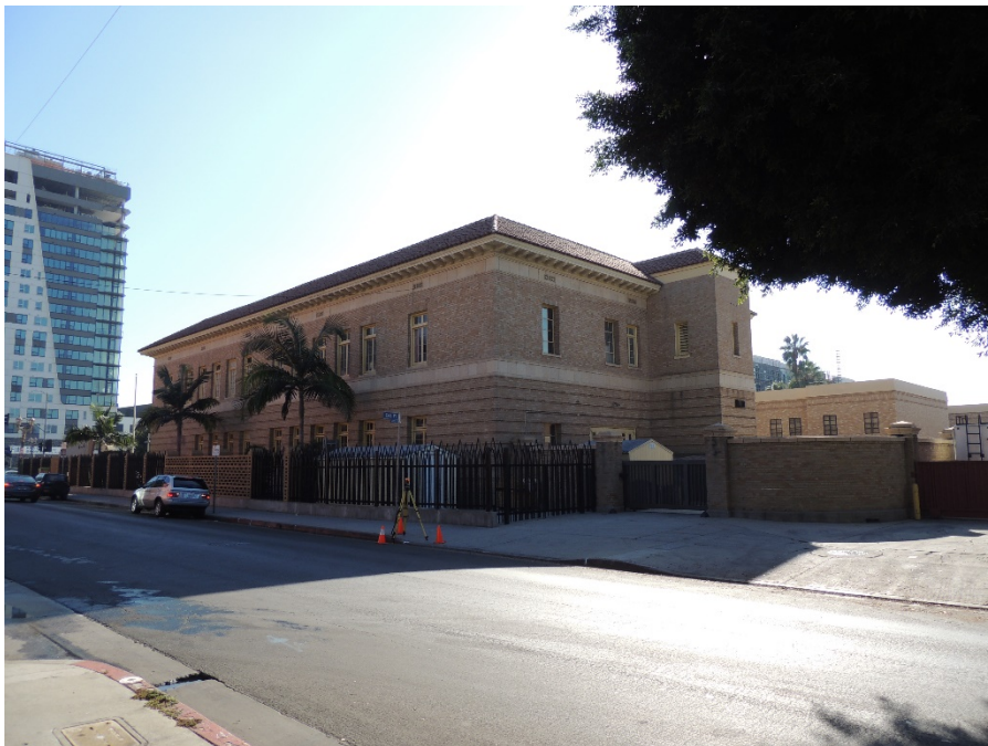
Fire Station No. 27, view facing southeast.
