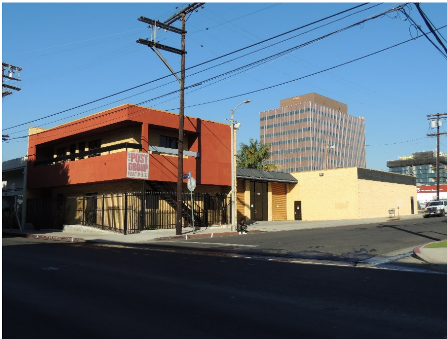
1413 N. Cole Avenue, view facing northwest.
