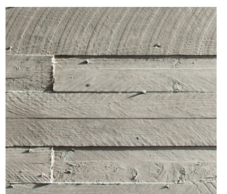
6. BOARD FORMED CONCRETE
