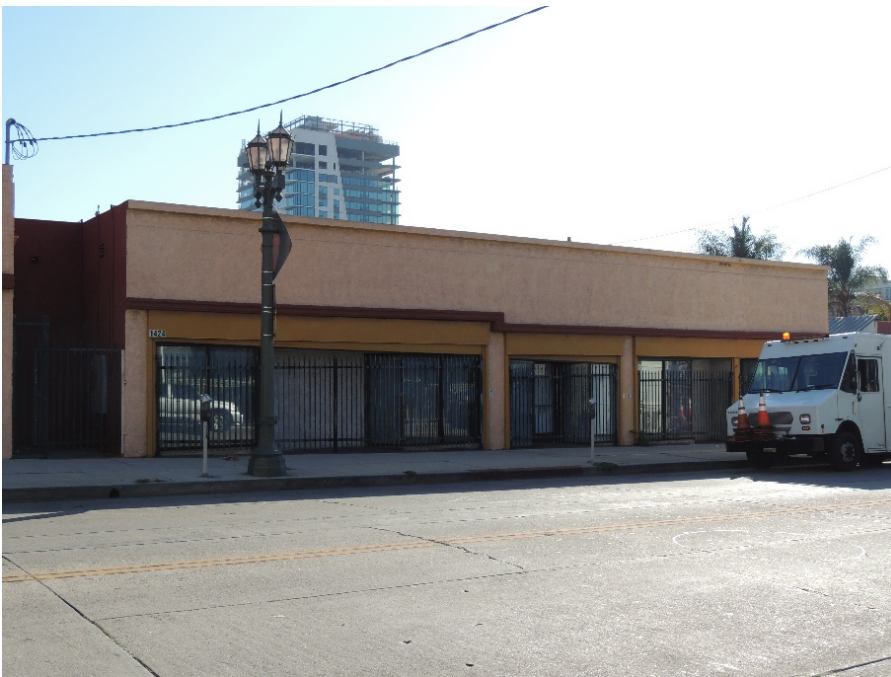
1424-1430 N. Wilcox Avenue, view facing southeast.
