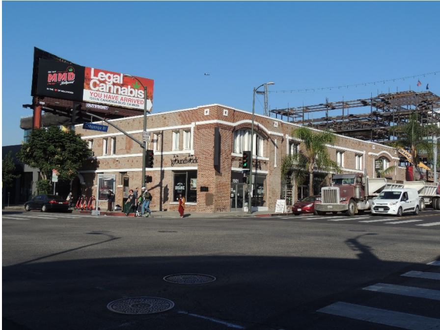
1501 N. Cahuenga Boulevard, view facing northwest.
