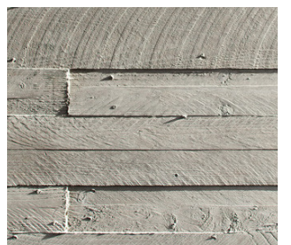
6. BOARD FORMED CONCRETE
