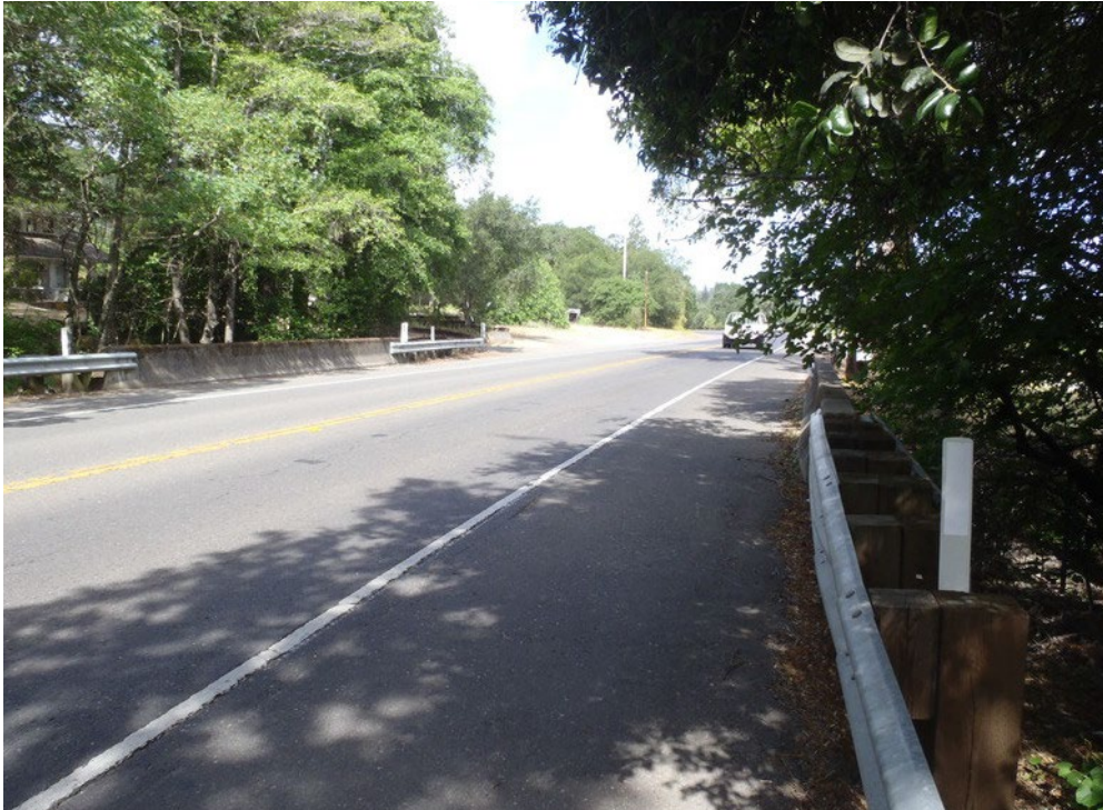
Figure 1-3 Northbound View of Existing Bridge
