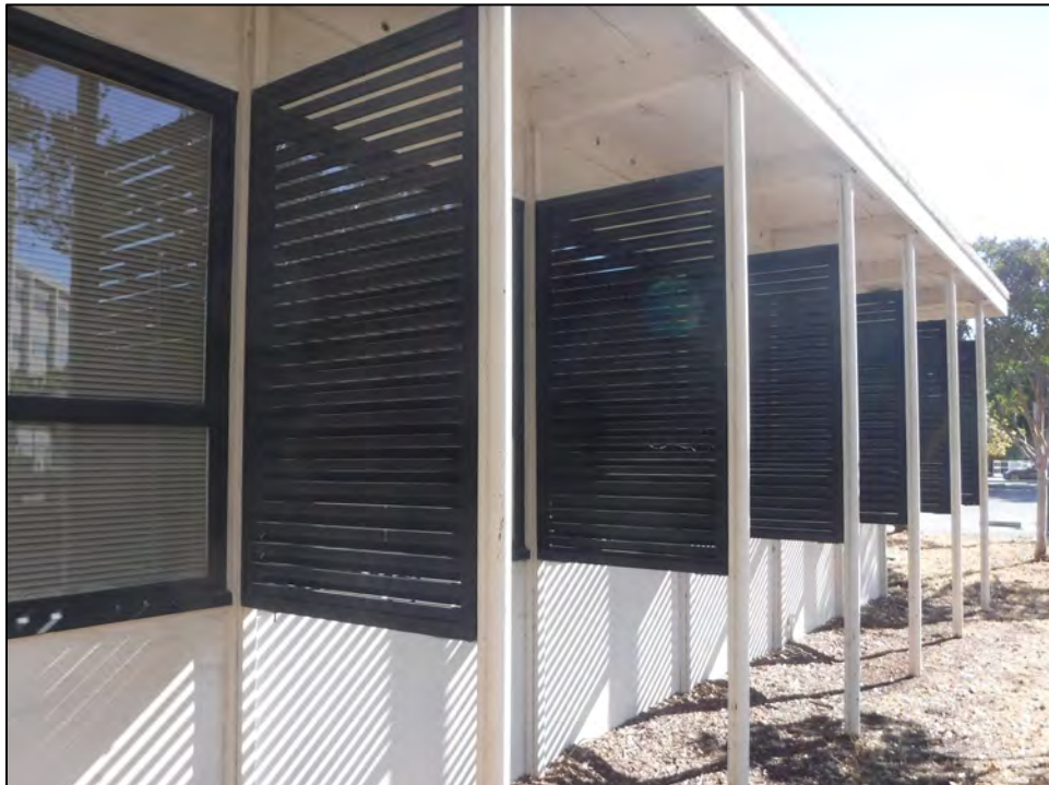
Photograph 3: Detail of windows and wood screens along façade, camera facing south, September 23, 2020.
