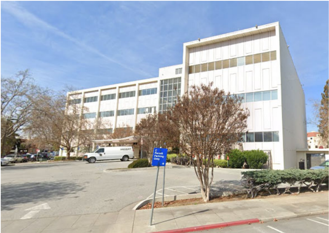
Photograph 2. Palo Alto Superior Courthouse, view to west from Grant Avenue
