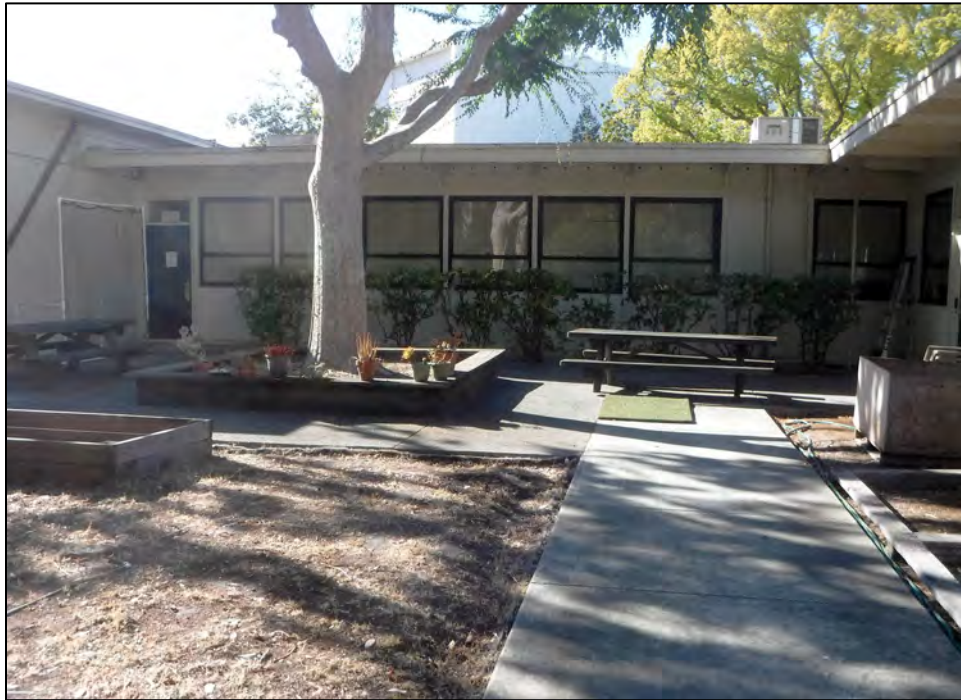
Photograph 8: View of rear courtyard, camera facing west, September 23, 2020.
