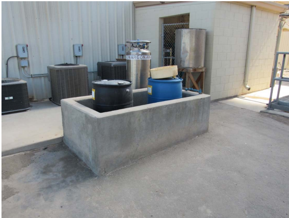
Photo 4: Looking at the secondary containment area at south side of the control building.
