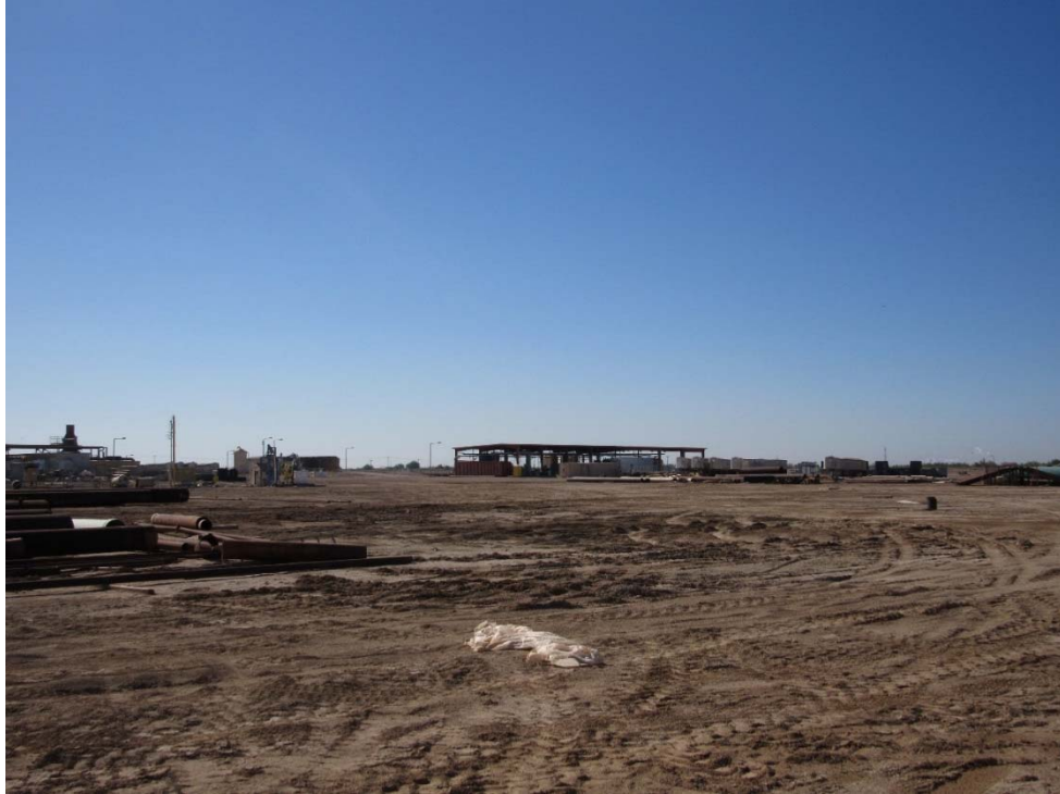
Photo 29: Looking southeast across the Plant Site from the northwest corner.
