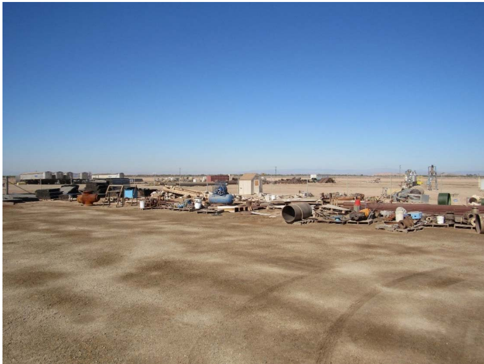
Photo 28: Looking southwest across the storage area of the Plant Site.
