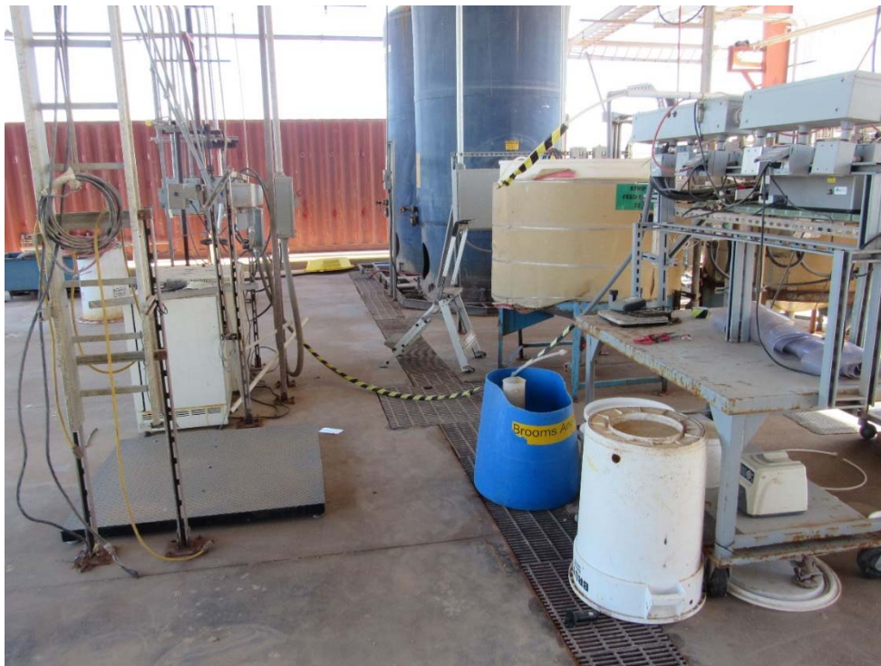
Photo 44: Looking at the north end of the ES Mineral Test area.
