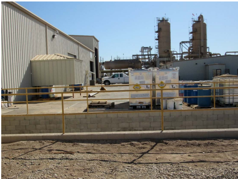
Photo 10: Looking at the 5-gallon buckets on the south side of the warehouse building.
