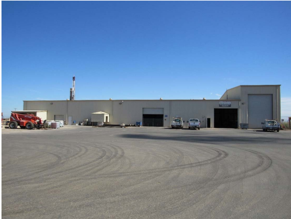
Photo 7: Looking north at the warehouse building.
