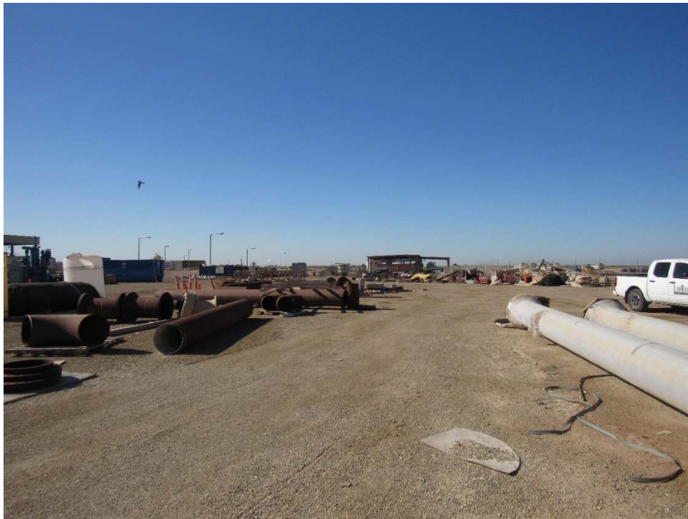
Photo 24: Looking south from the storage area of the Plant Site.
