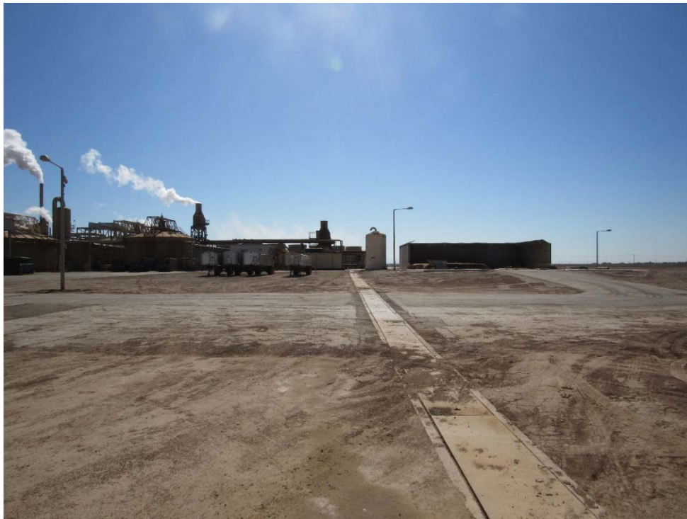
Photo 46: Looking east along the trench from the ES Mineral Test area toward the brine pond.
