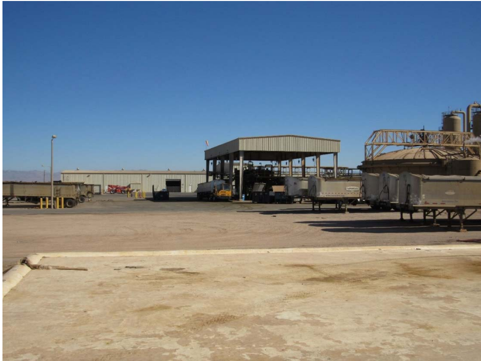
Photo 66: Looking at the belt filter area with trailer being loaded.
