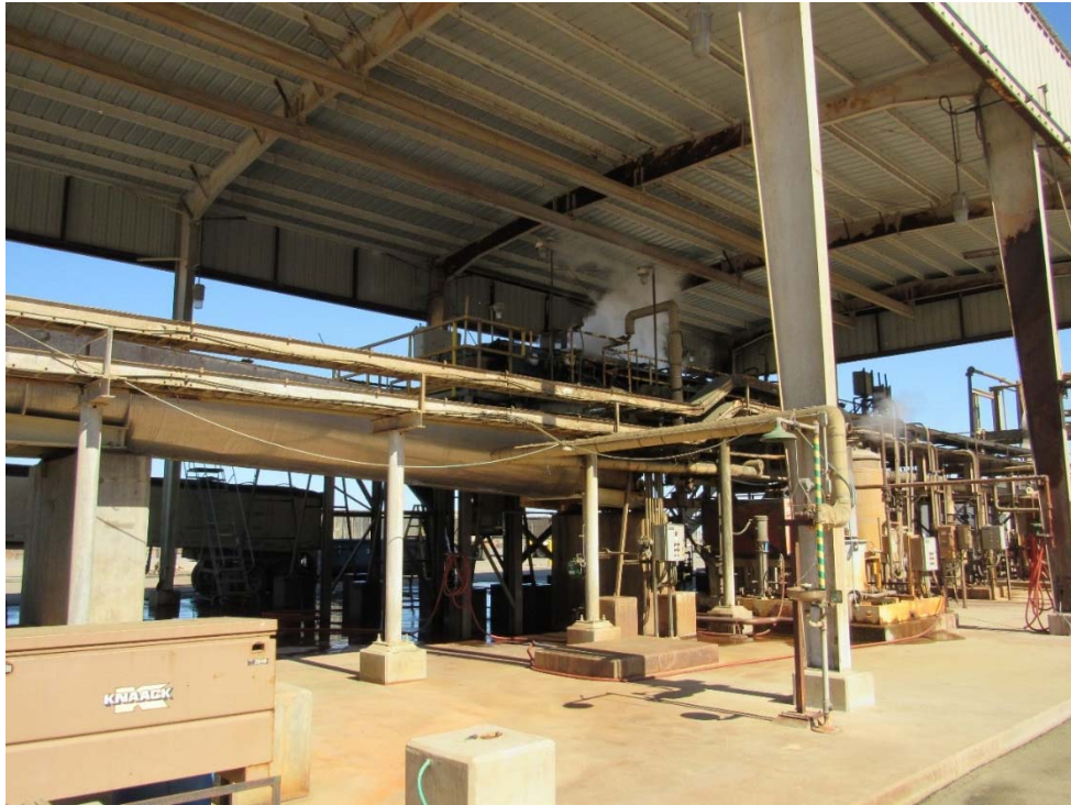
Photo 68: Looking within the belt filter area.
