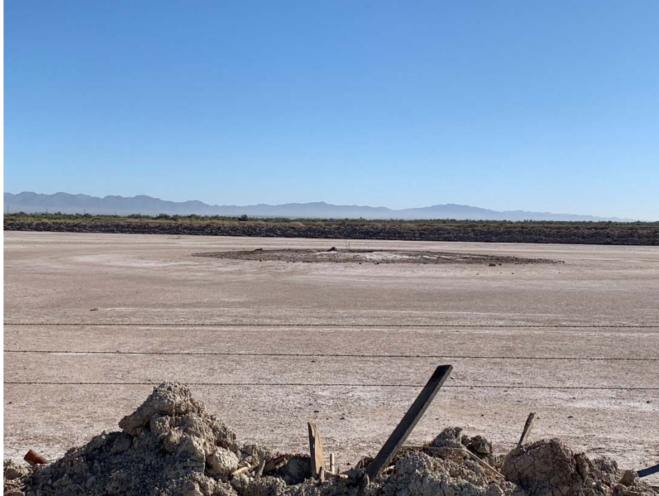
Photo 101: Looking at an abandoned carbon dioxide well at the northwest corner of the subject property.
