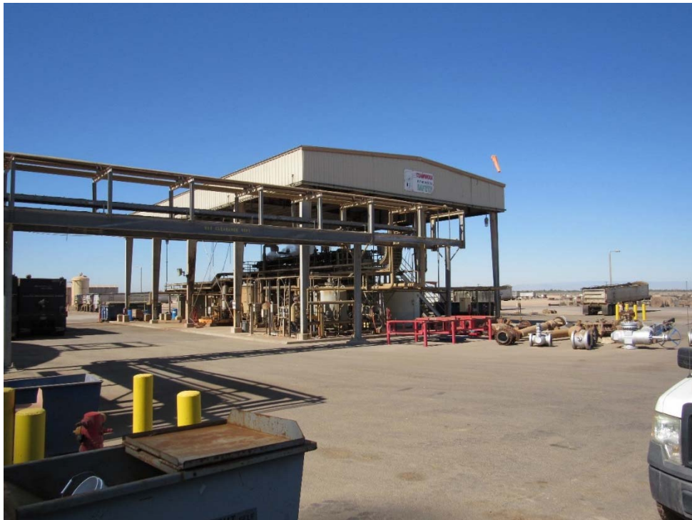
Photo 6: Looking southwest toward the belt filter area.
