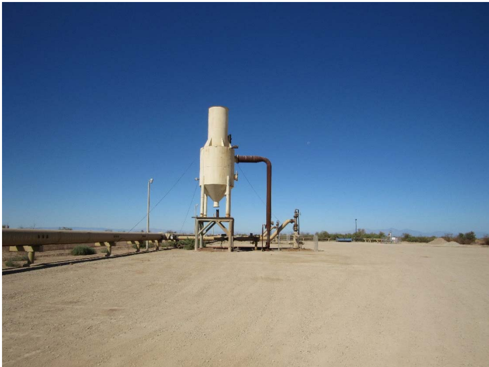
Photo 82: Looking west at the northeast well pad along the east boundary of the subject property.
