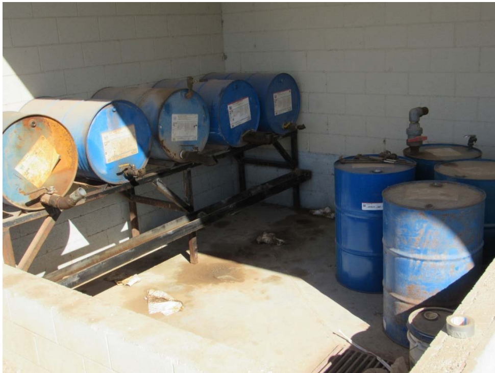
Photo 14: Looking at the oil staining within the secondary containment.
