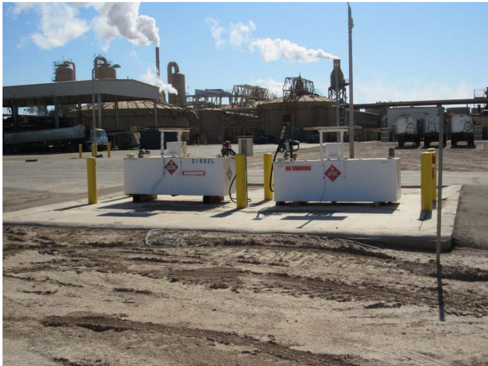
Photo 36: Looking at diesel and gasoline fuel tanks and pumps located just northeast of the ES Mineral Test area within the Plant Site.
