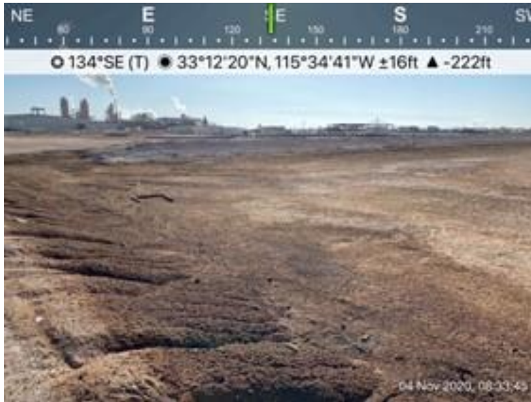
Figure 2: View of water retention basin with HR1 in background, facing east/southeast.
