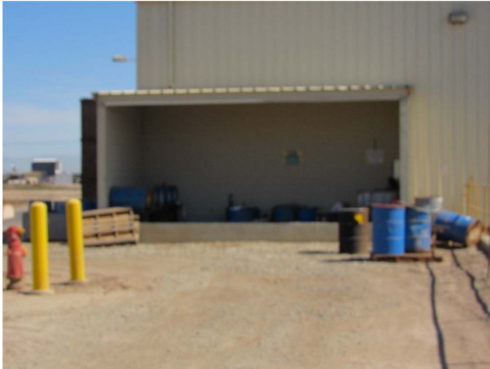
Photo 11: Looking at the secondary containment area at the southwest corner of the warehouse building.
