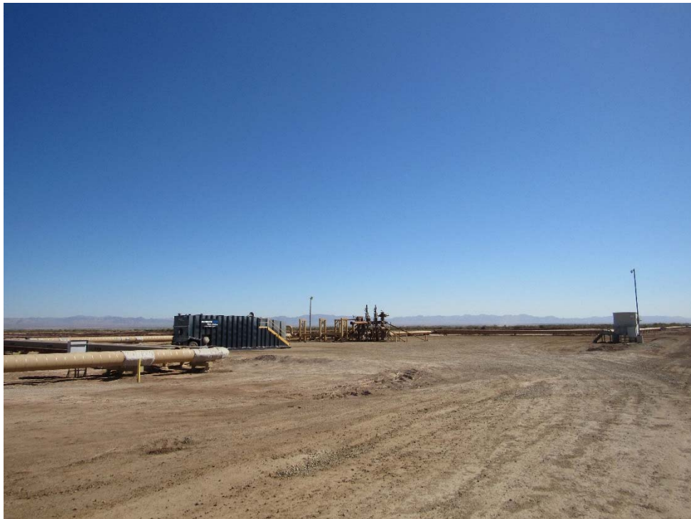
Photo 76: Looking at the southeast well pad just north of the northeast corner of the Geothermal Plant Facility.
