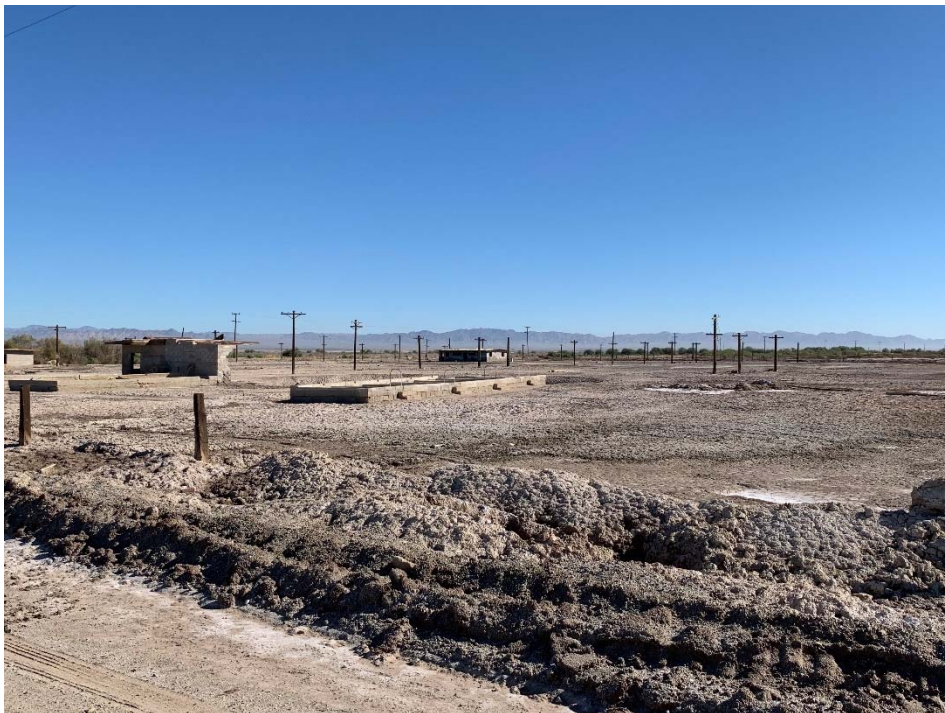
Photo 104: Looking south along the west boundary of the subject property.
