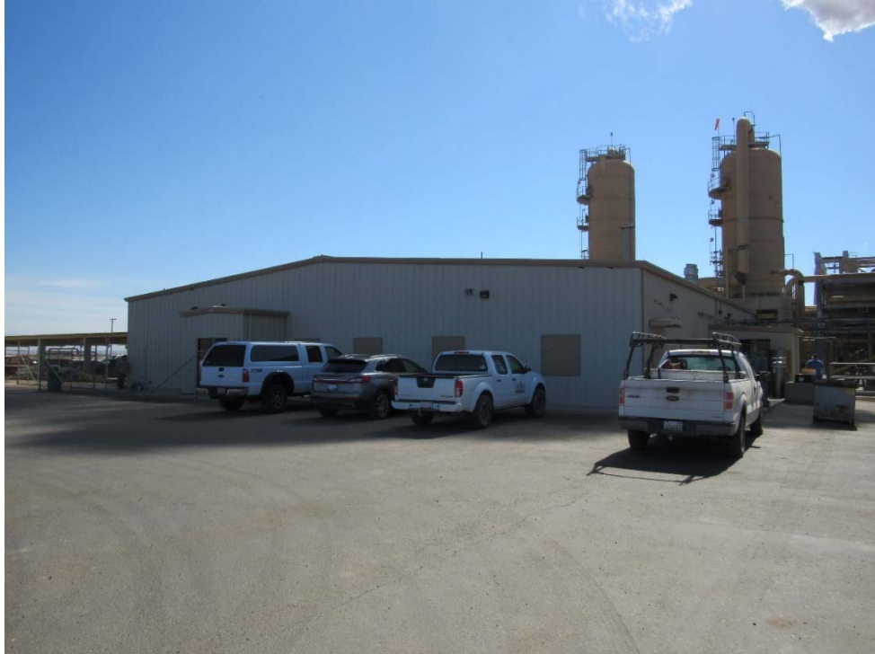
Photo 1: Looking east/northeast at the west side of the control building.
