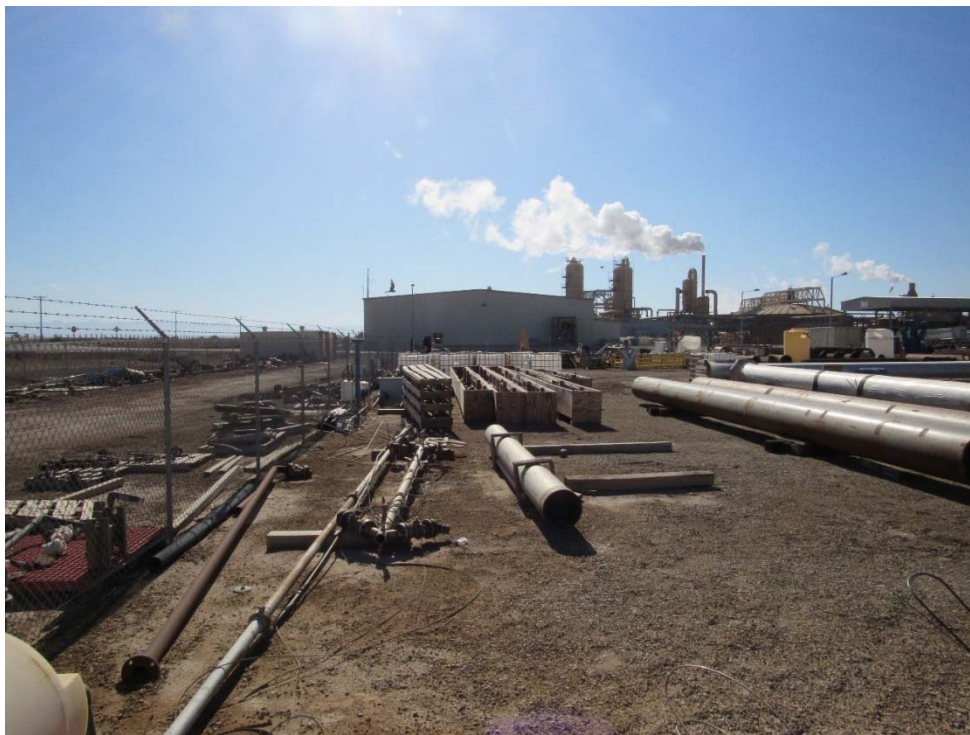
Photo 22: Looking east toward the warehouse building from the storage area of the Plant Site.
