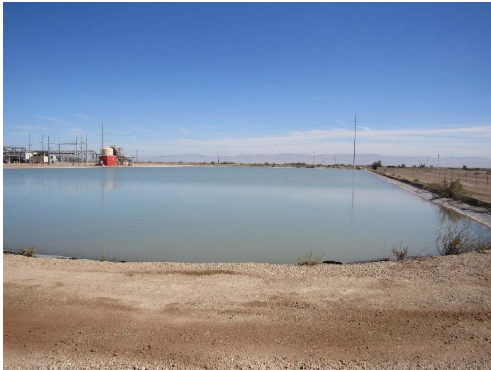
Photo 52: Looking north at the make-up water pond located in the northeast corner of the Plant Site.
