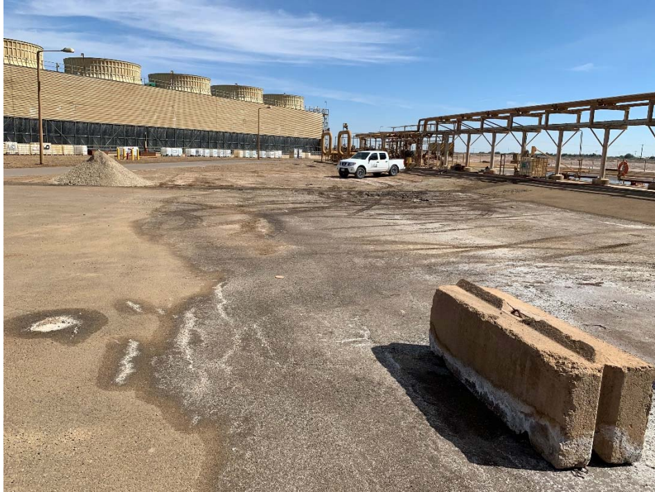
Photo 58b: 10/16/19 spillage shown in photo 58a was within asphalt containment area, the liquid drained to the sump and pumped back to brine pond.
