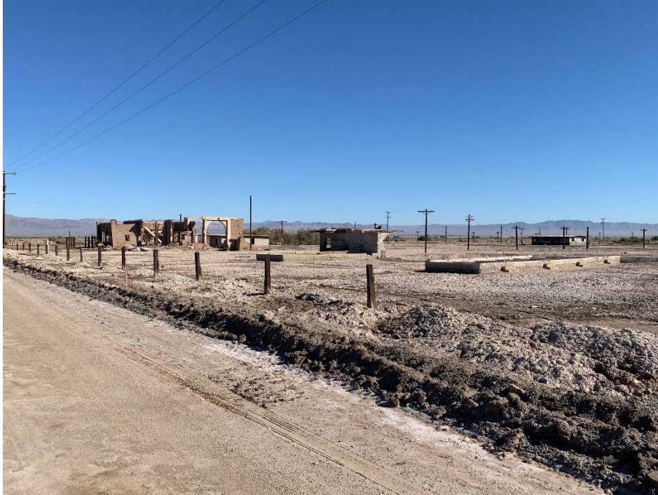
Photo 105: Looking south along the west boundary of the subject property.
