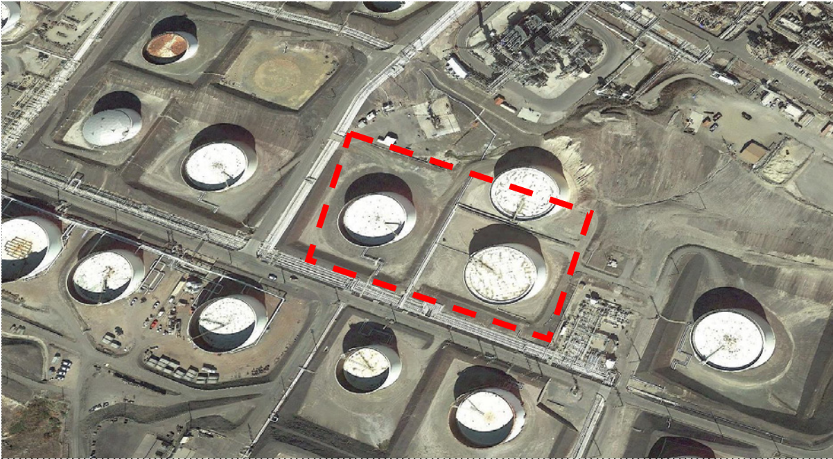
Figure 4.2-13 Existing Use and Future Location of Pre-Treatment Unit at Rodeo Site
