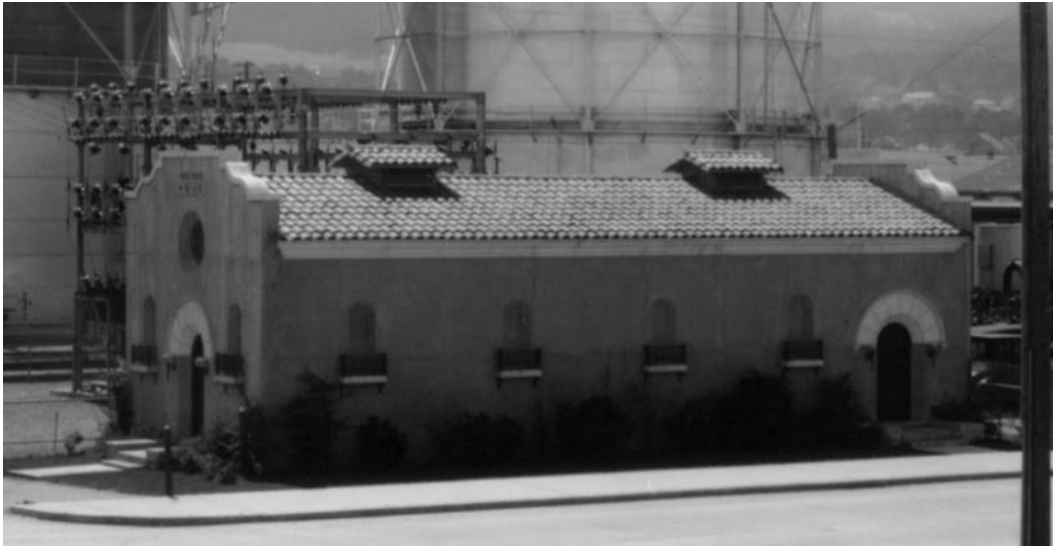
Figure 15. Excerpt from 1929 photograph depicting the primary (eastern) and secondary (northern) elevations of the former substation at 498 Del Monte Avenue.
