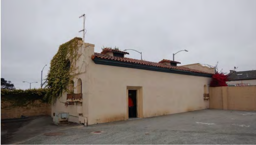
Figure 3. Western and southern elevations of 498 Del Monte Avenue, which was built in 1926. Notice the walls that abut the building at the right and left. View looking northeast
