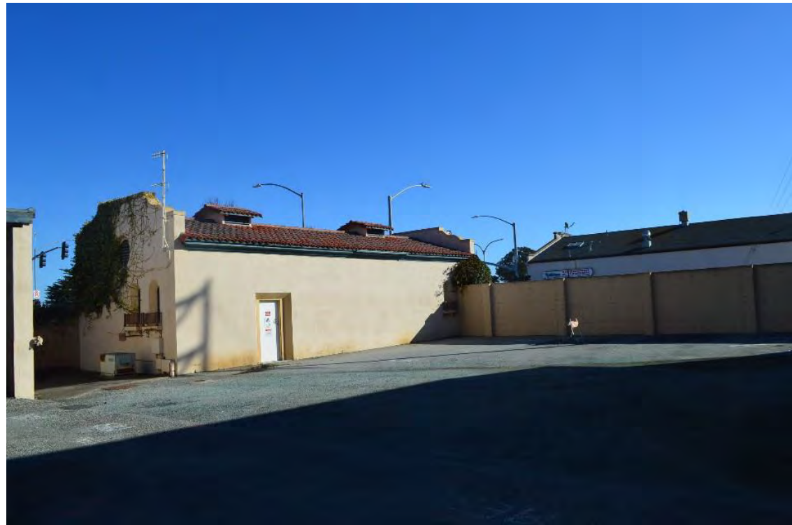
Control Building (to be excluded from excavation area) and interior of eastern perimeter wall where driveway to be constructed, view from southwest
