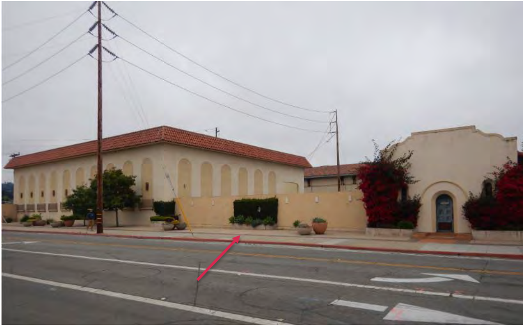
Figure 7. Photograph depicting the eastern wall that encloses the parcel at center; a portion of this wall will be removed for the installation of a new gate (denoted by red arrow). 498 Del Monte Avenue is at right, and the tall walls that border the substation electrical transmission equipment to the north (at center) and east (at left) also are visible. View looking west-southwest from Figueroa Street.
