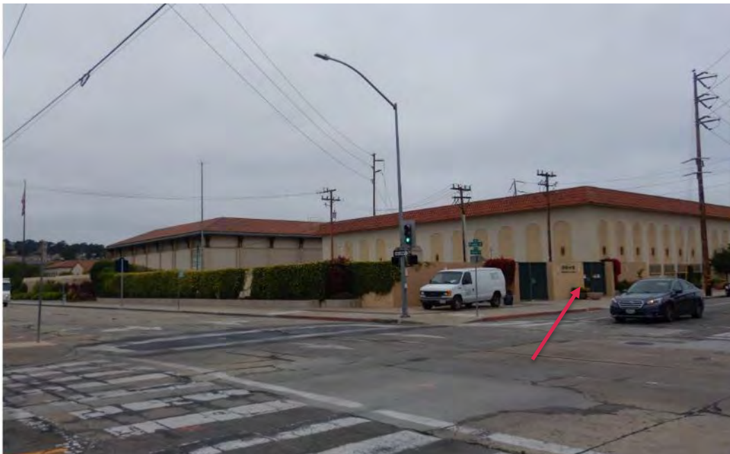
Figure 8. View of wall that encloses parcel (in foreground). The gate that will be enlarged as part of the proposed project is denoted with a red arrow. The tall walls that border the substation electrical transmission equipment to the east (at right) and south (at center) as well as a portion of the Monterey Sports Complex (at left) also are visible. View looking northeast from the intersection of Figueroa and East Franklin streets.
