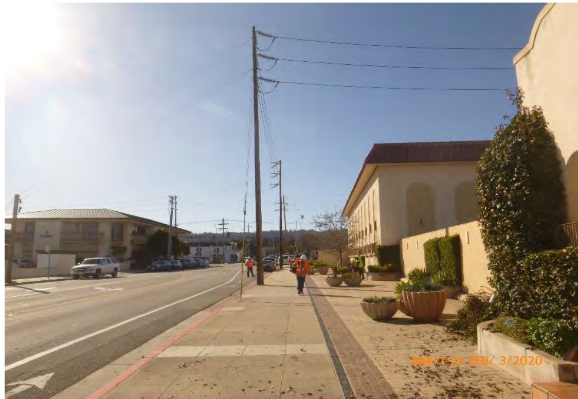
Eastern perimeter walls of Project Site on Figueroa Street, view to south towards East Franklin Street (driveway to be constructed beyond planter box in foreground)
