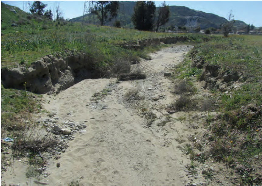
View looking south within Drainage B (see Picture Point 1).
