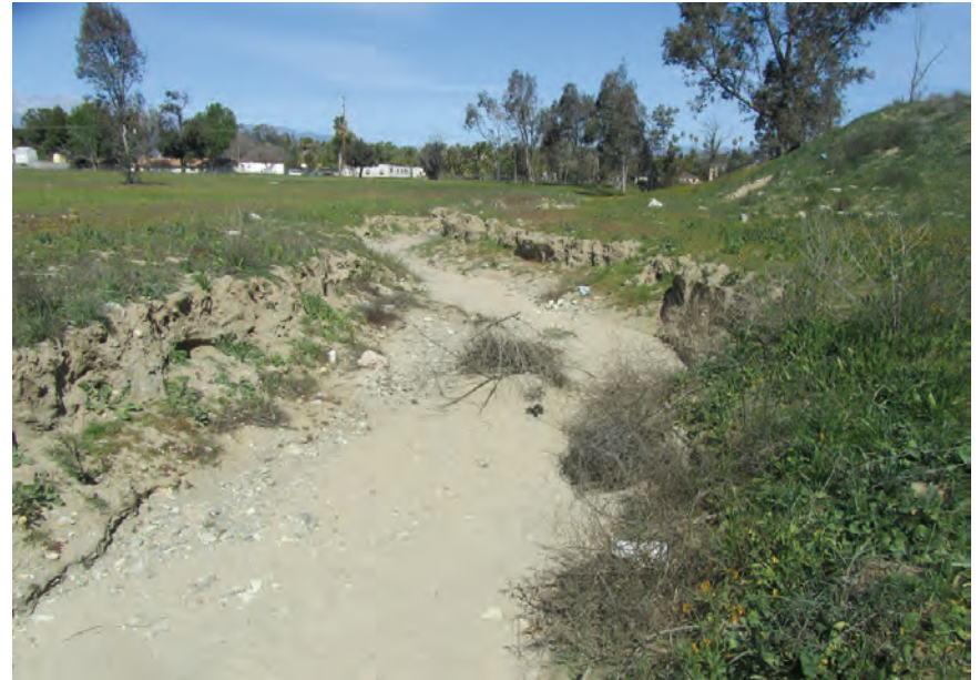
View looking north within Drainage B (see Picture Point 2).
