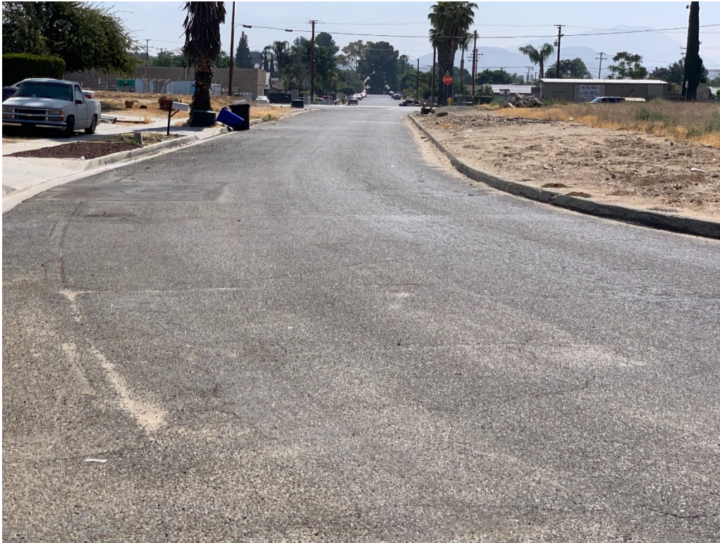
Photograph 5: Storm drain alignment within existing road.
