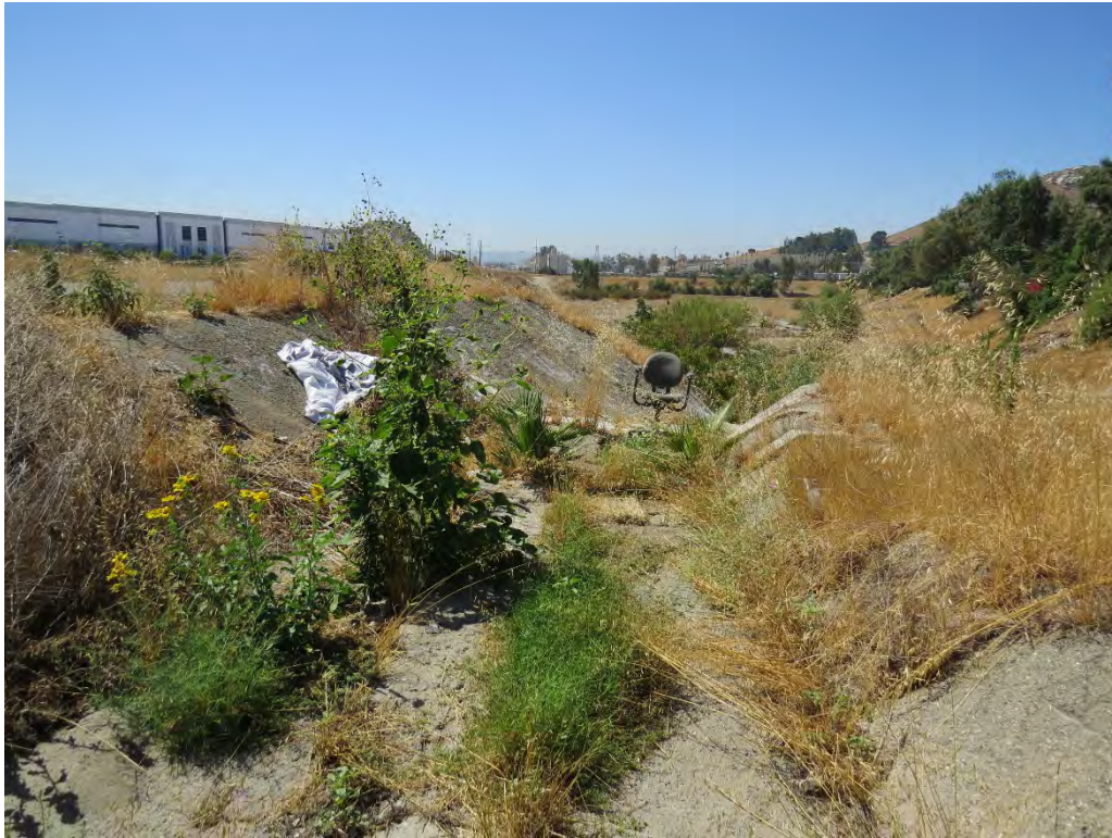
Photograph 3: Non-native vegetation growing in the concrete lined v-ditch that enters the northern portion of the basin.
