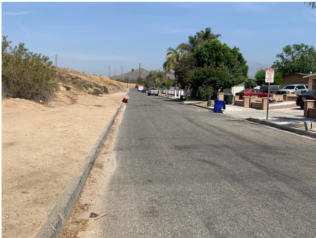
Photograph 4: Storm drain alignment in existing road.
