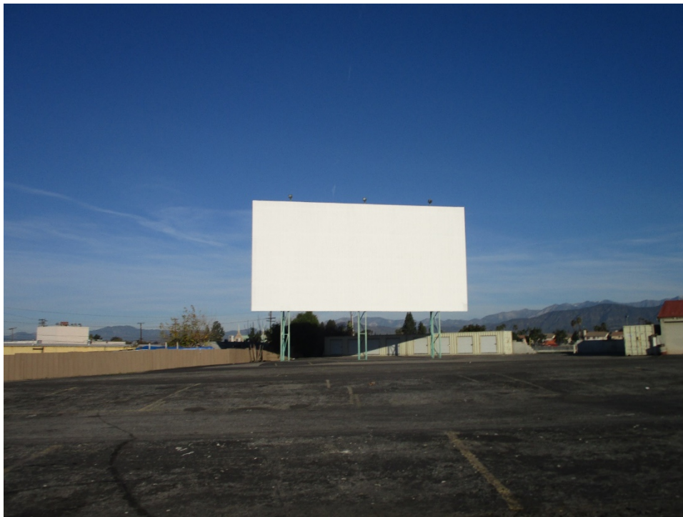
Figure 5. Screen 4, main elevation, view looking northwest (IMG_3102)
