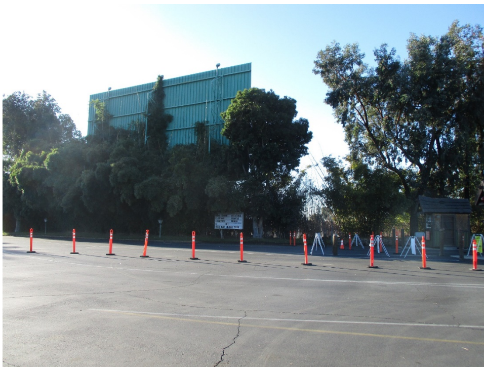
Figure 6. Screen 1, rear elevation, view looking southeast (IMG 3081)
