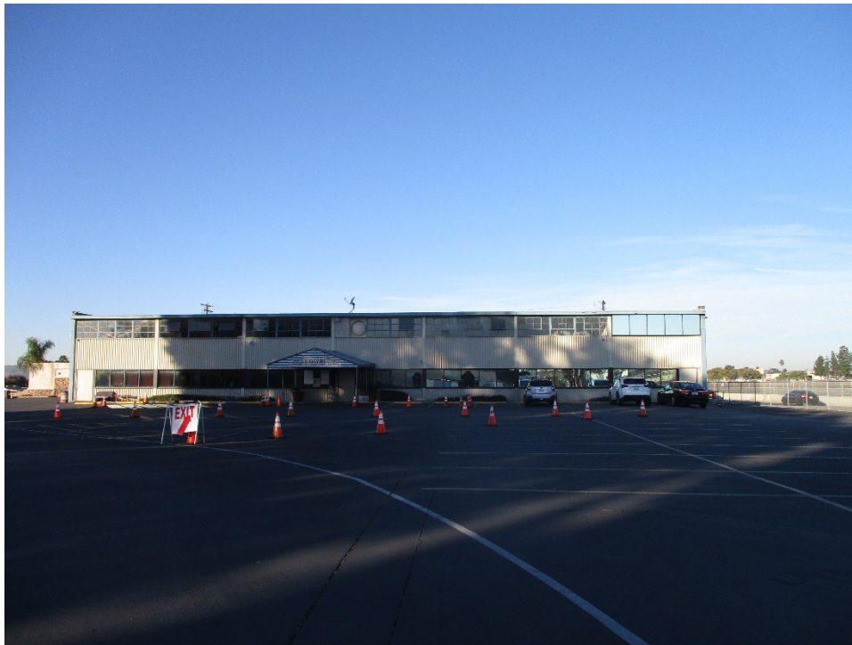
Figure 3. Office: main elevation, view looking west (IMG 3078)
