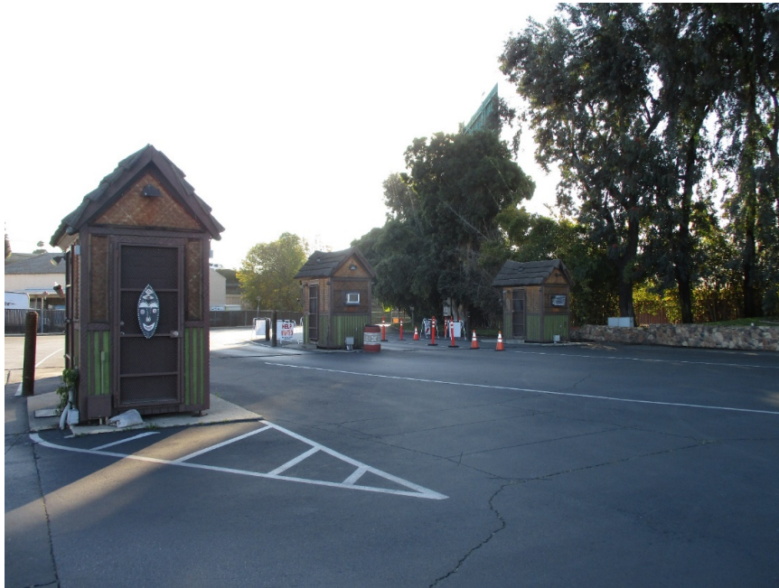
Figure 8. Three ticket booths, view looking east (IMG 3079)
