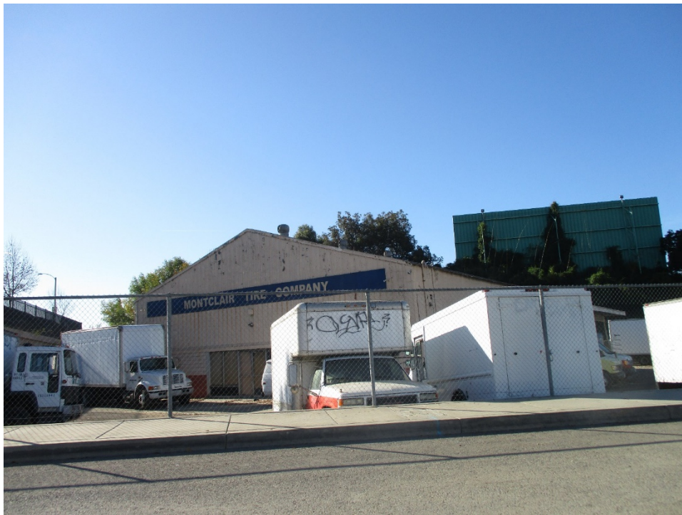
Figure 2. Montclair Tire Company: main and northeast elevations, view looking south (IMG 3167)
