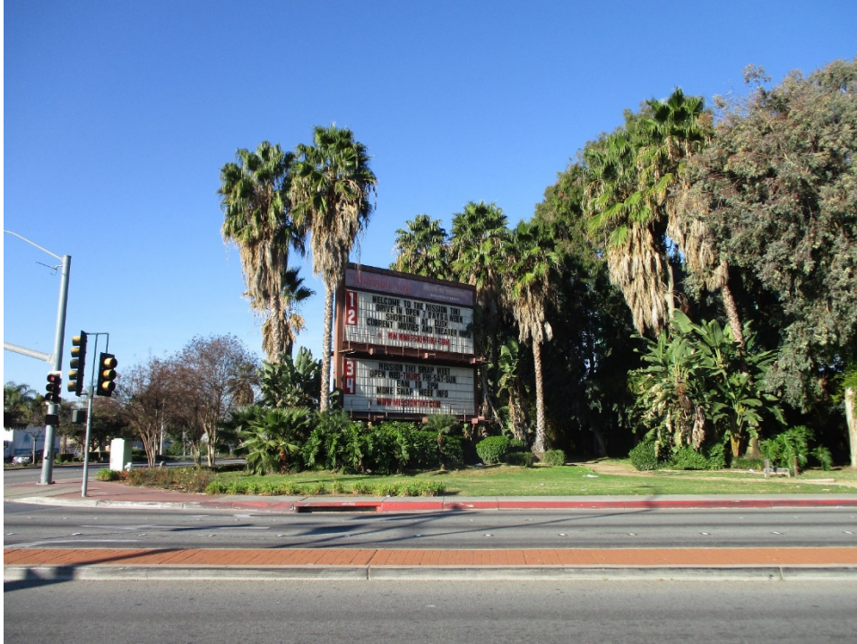
Figure 7. Marquee structure at the corner of Ramona Avenue and Mission Boulevard, view looking west (IMG 3146)
