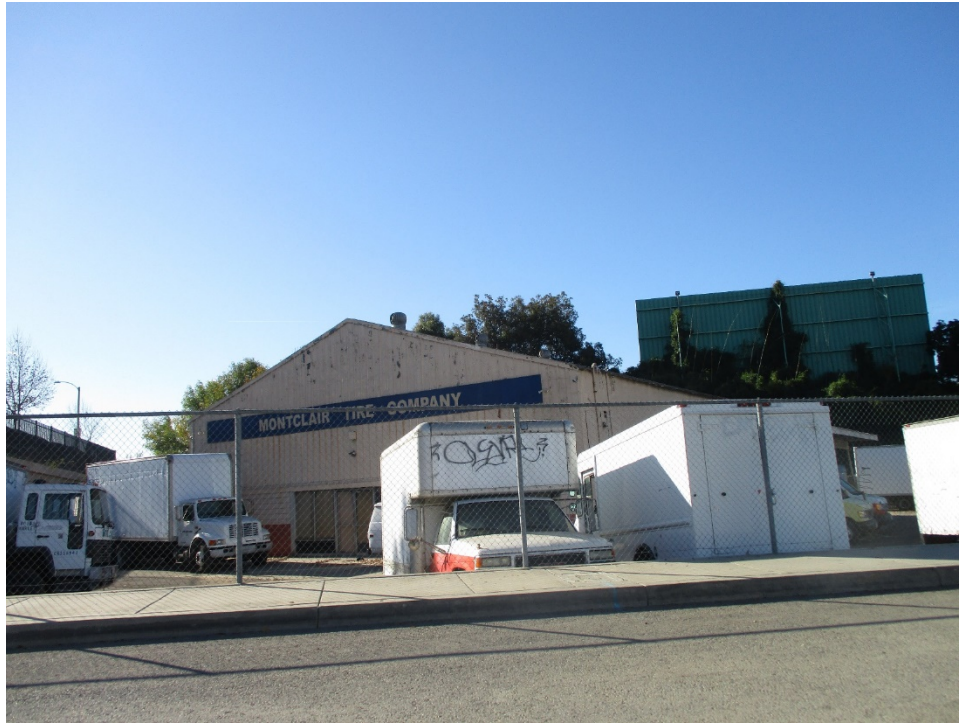
Figure 18. Montclair Tire Company: main and northeast elevations, view looking south (IMG 3167)
