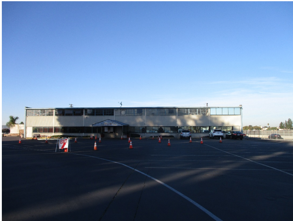
Figure 9. Office: main elevation, view looking west (IMG 3078)
