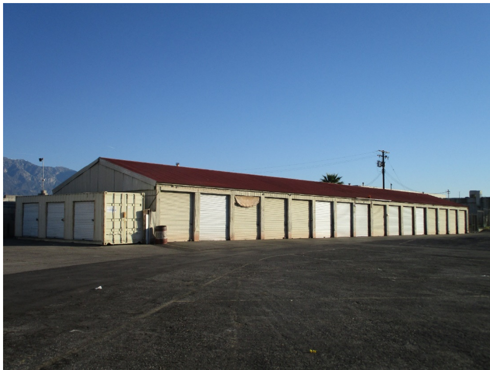
Figure 10. Screen 4, main elevation, view looking northwest (IMG_3103)
