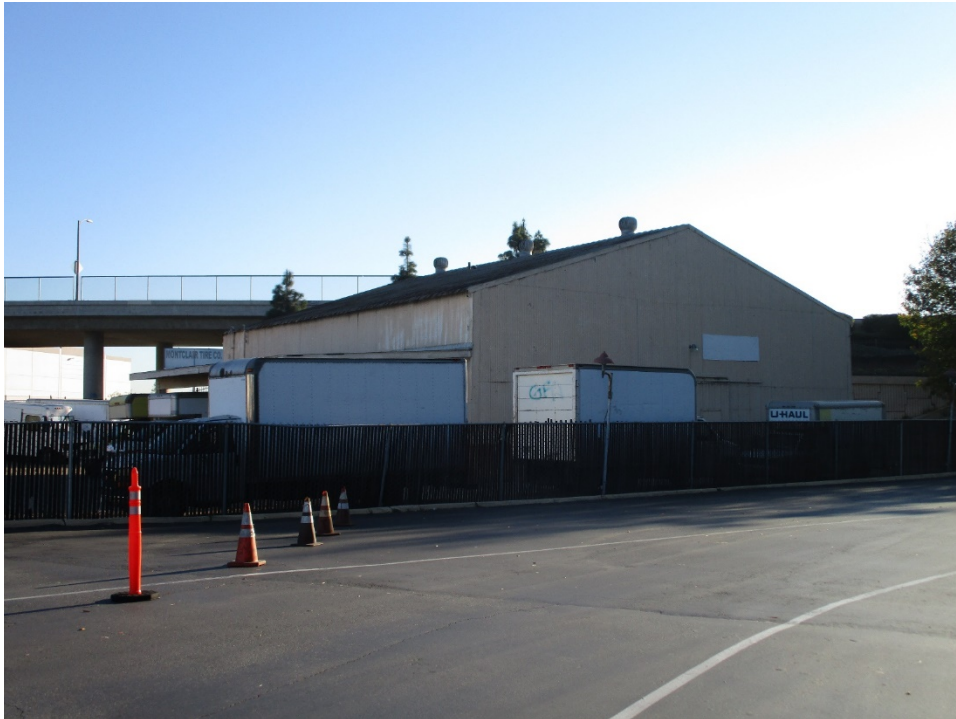
Figure 1. Montclair Tire Company: main and southwest elevations, view looking east (IMG 3118)
