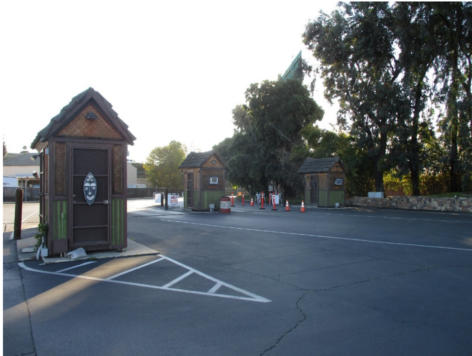
Figure 14. Three ticket booths, view looking east (IMG 3079)
