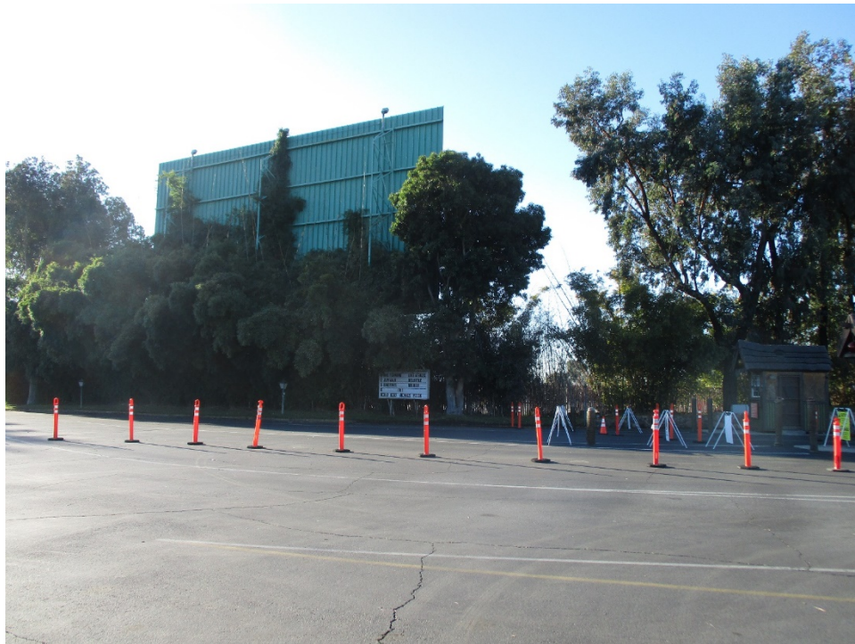
Figure 12. Screen 1, rear elevation, view looking southeast (IMG 3081)
