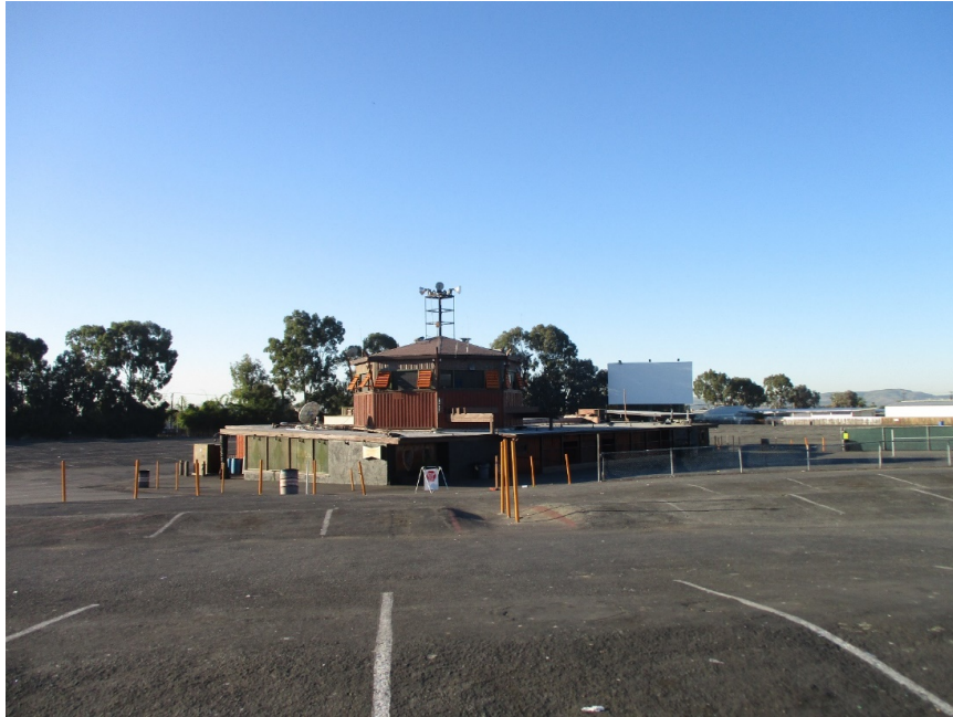
Figure 1. Projection Building/Snack Bar: north and east elevations, view looking southwest (IMG 3089)
