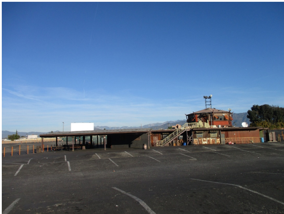
Figure 8. Projection Building/Snack Bar: south (main) elevation, view looking north (IMG 3095)
