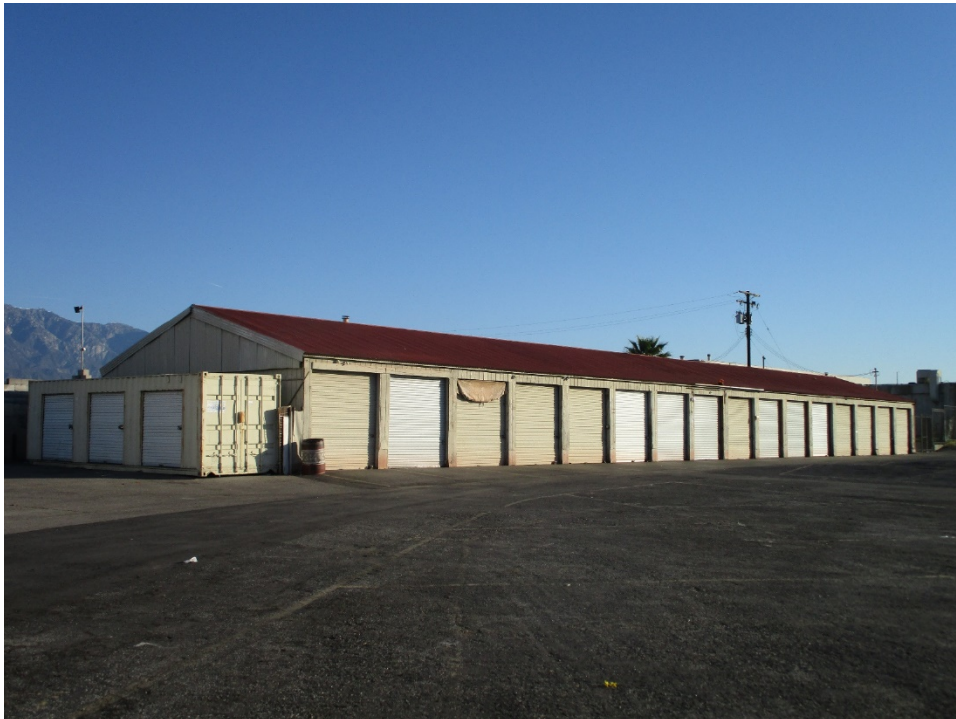
Figure 4. Screen 4, main elevation, view looking northwest (IMG_3103)
