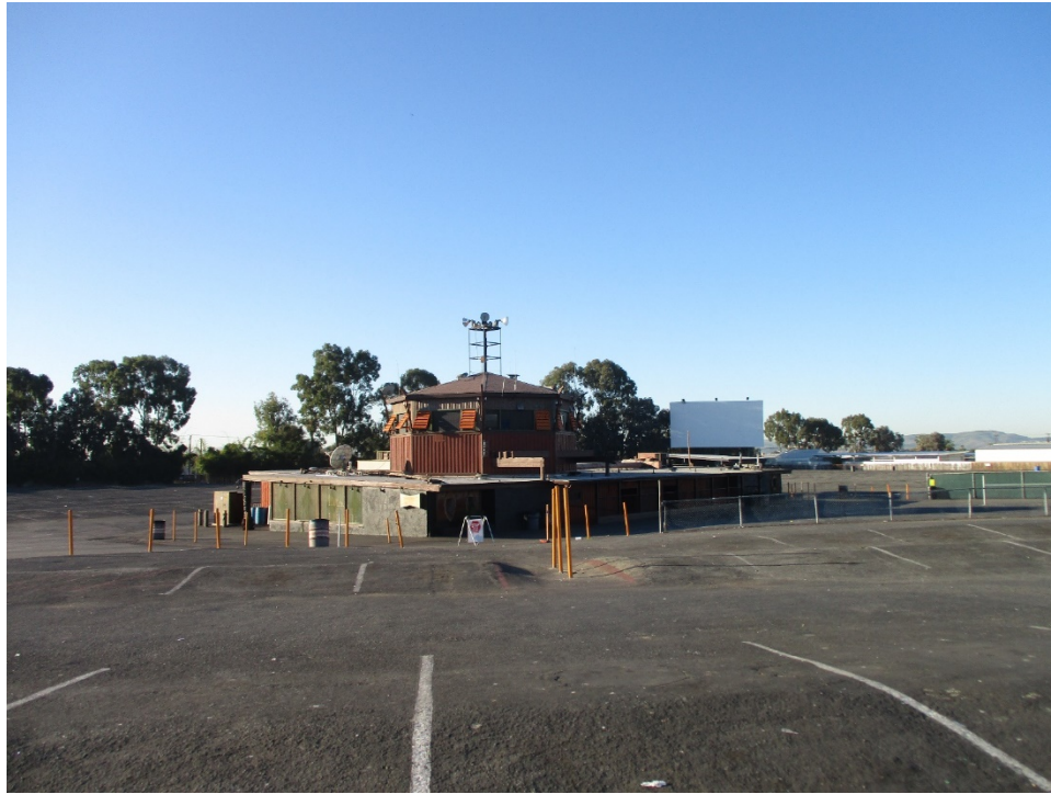
Figure 7. Projection Building/Snack Bar: north and east elevations, view looking southwest (IMG 3089)
