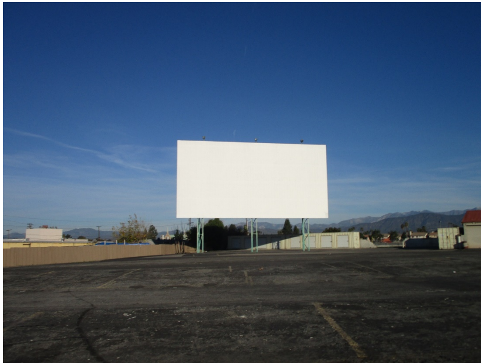
Figure 11. Screen 4, main elevation, view looking northwest (IMG_3102)
