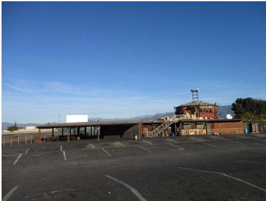
Figure 2. Projection Building/Snack Bar: south (main) elevation, view looking north (IMG 3095)
