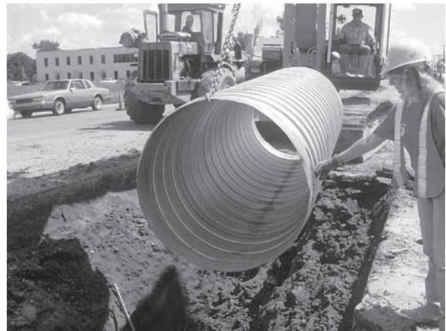
Reduced excavation because of ULTRA FLO's smaller outside diameter.
