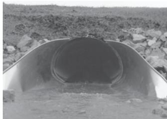
End Sections are available for CSP Pipe-Arch
