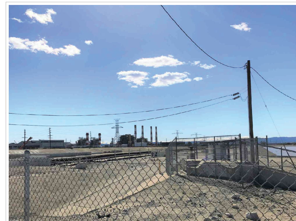
Photo D - View looking south toward the project site from Glenoaks Boulevard, east of the Hansen Spreading Grounds, approximately 0.52-mile north of the project site.
