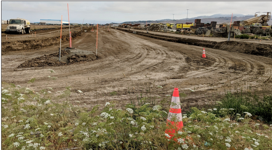
Photograph 3: View of the under construction segment of Devlin Road.
