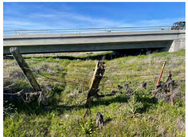
The north end of Wetland W3 before going off site and under the newly constructed bridge.
