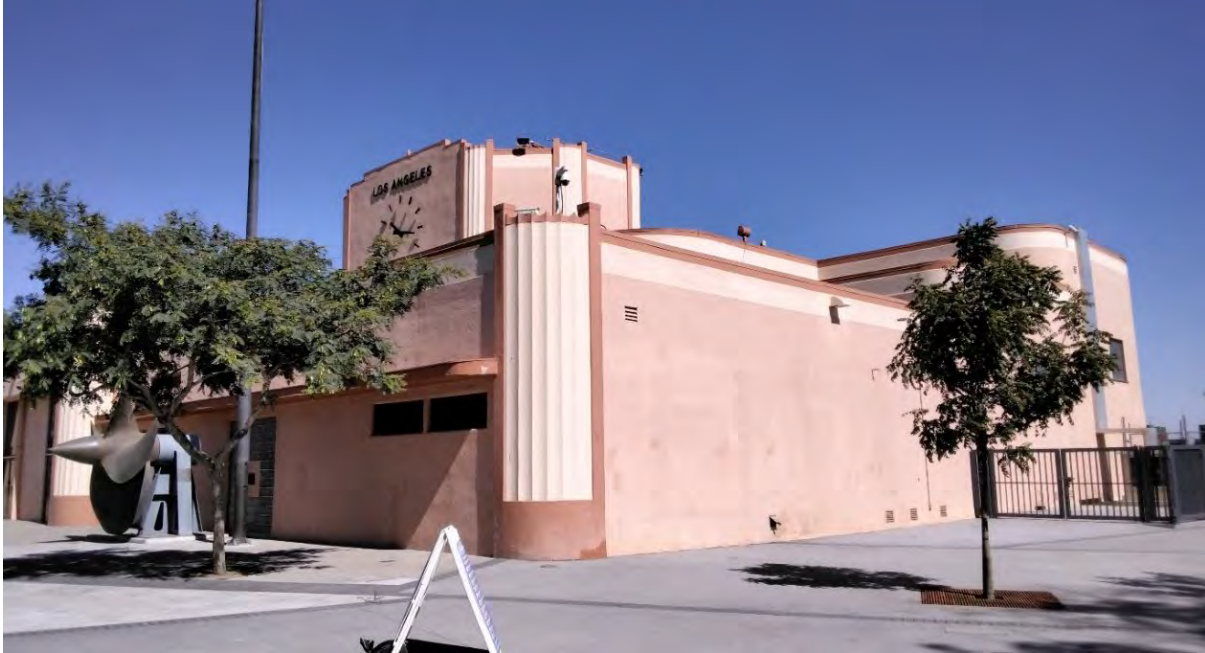
Figure 16 South and West Elevations of the San Pedro Municipal Ferry Building, Facing Northeast
