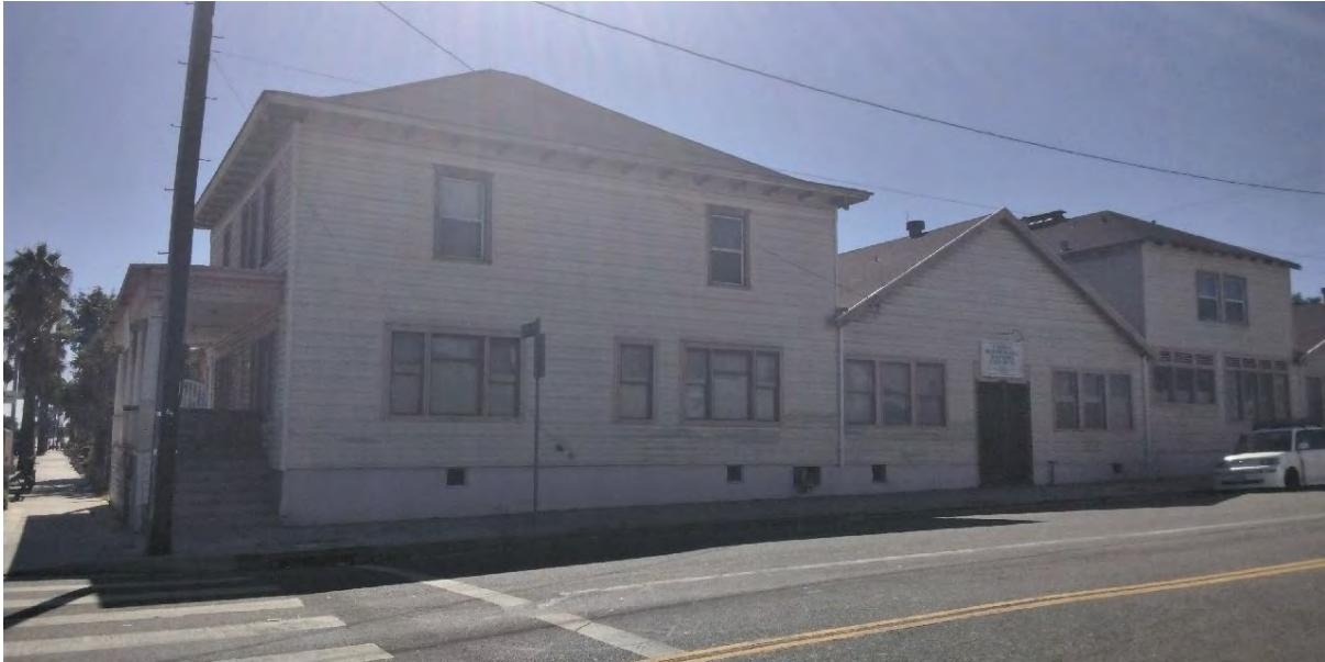
Figure 19 Secondary Elevation of 101 South Harbor Boulevard (Senator William H. Savage House), Facing South
