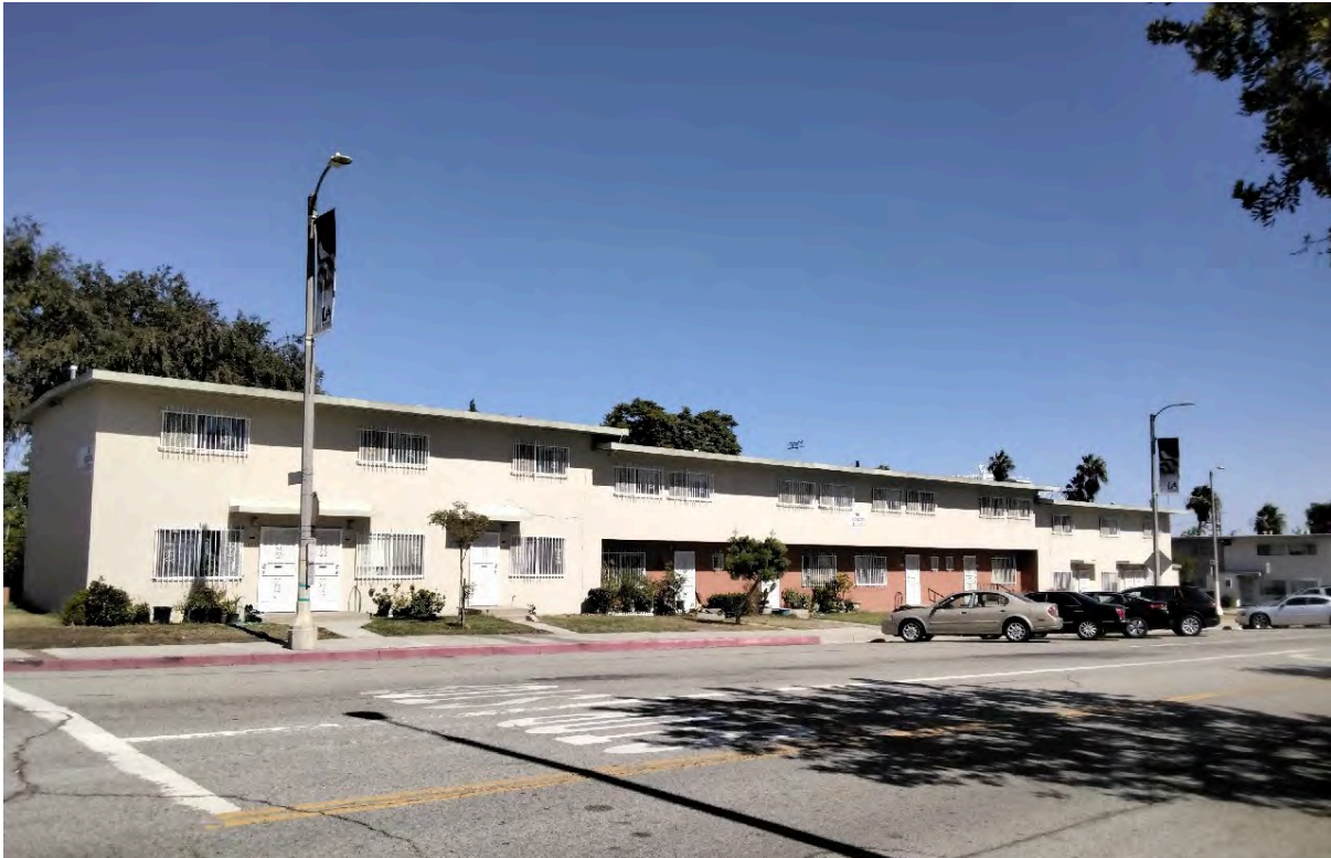
Figure 11 Portion of RSP Complex along West 1st Street, Facing Southeast
