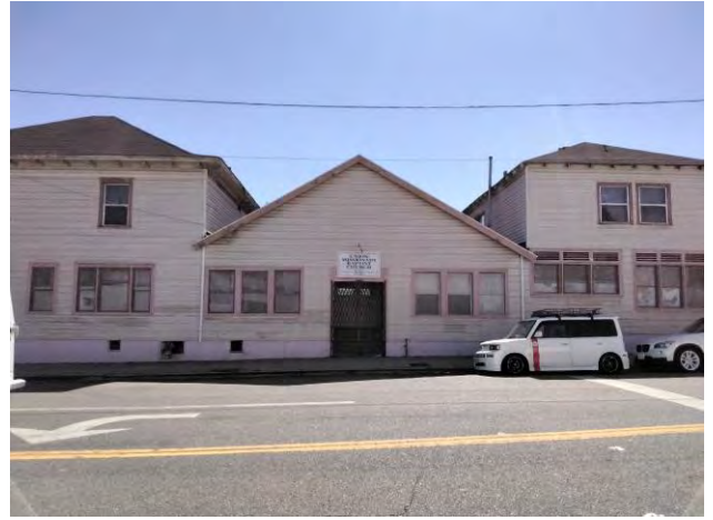
North elevation depicting additions and West 1st Street entrance; view south
