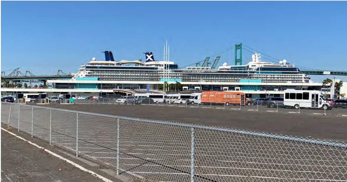
Figure 17 South Elevation of the Los Angeles Cruise Terminal, Facing North
