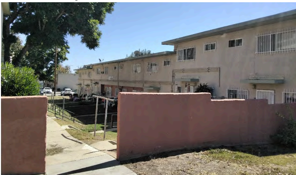
Figure 10 Portion of RSP Complex along South Mesa Street between West 1st Street and West 2nd Street, Facing Southeast
