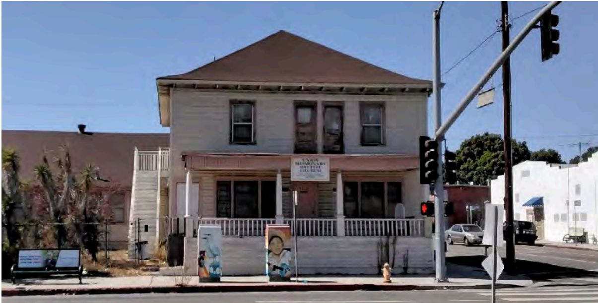
Figure 18 Primary Elevation of 101 South Harbor Boulevard (Senator William H. Savage House), Facing West
