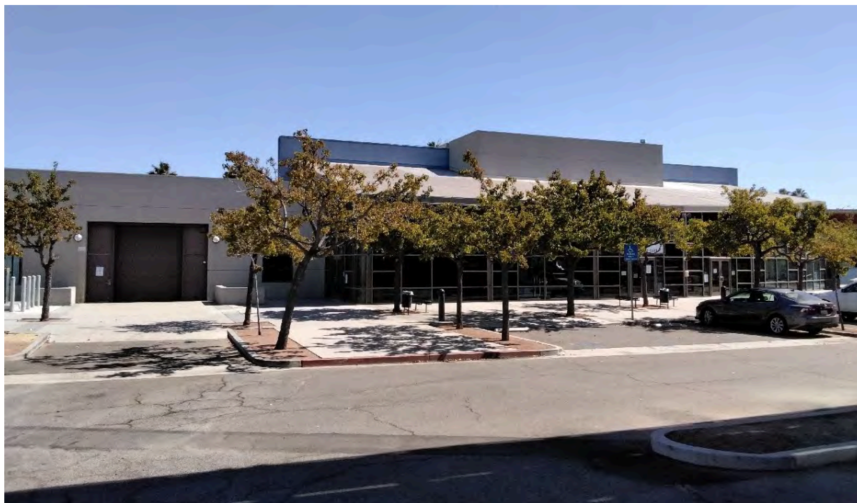
Figure 25 West Elevation of Boys and Girls Club Building, Facing East
