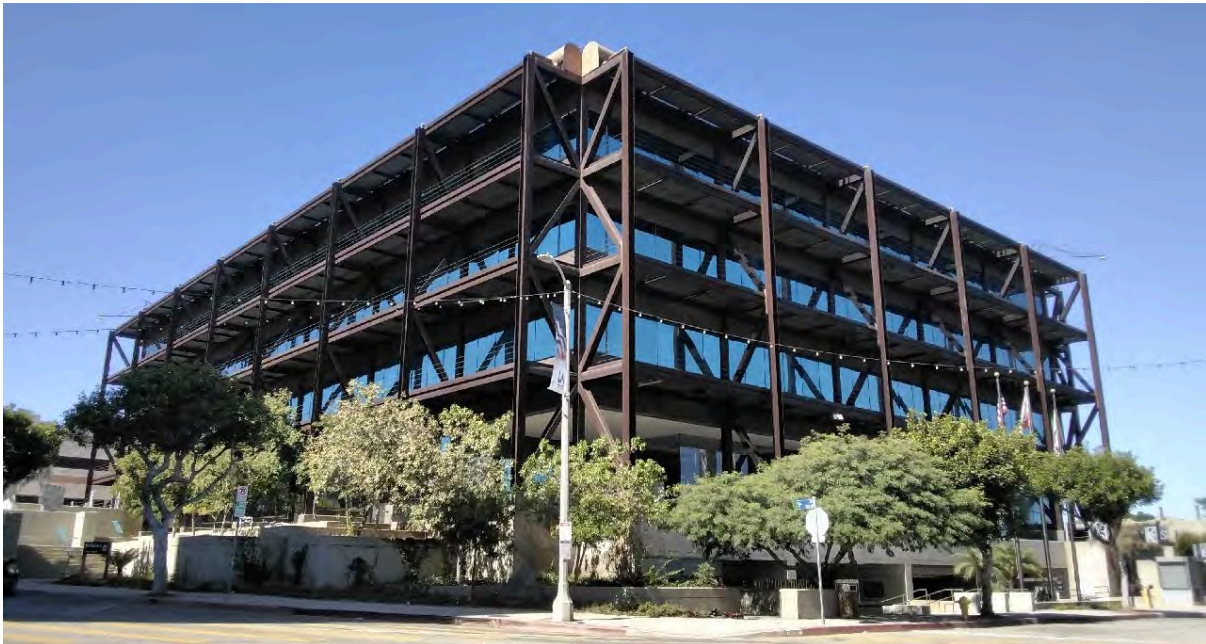
Figure 22 South and East Elevations of the POLA Administration Building, Facing Northwest
