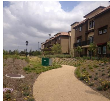
Underground Cistern Taylor Yard
