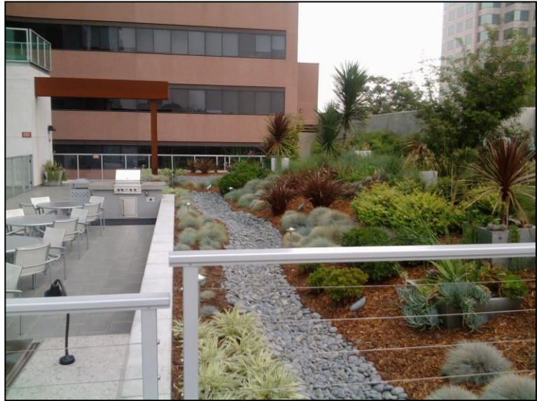
Bioretention (Planter Boxes) Watermarke Tower
