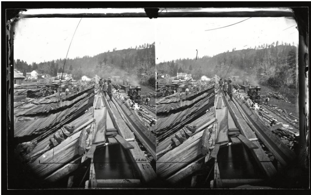
**Exhibit 1.** An early photograph of the Felton Flume (center) alongside the narrow gauge Santa Cruz and Felton Railroad (engine and tracks at right) (University of California, Santa Cruz Special Collections).
