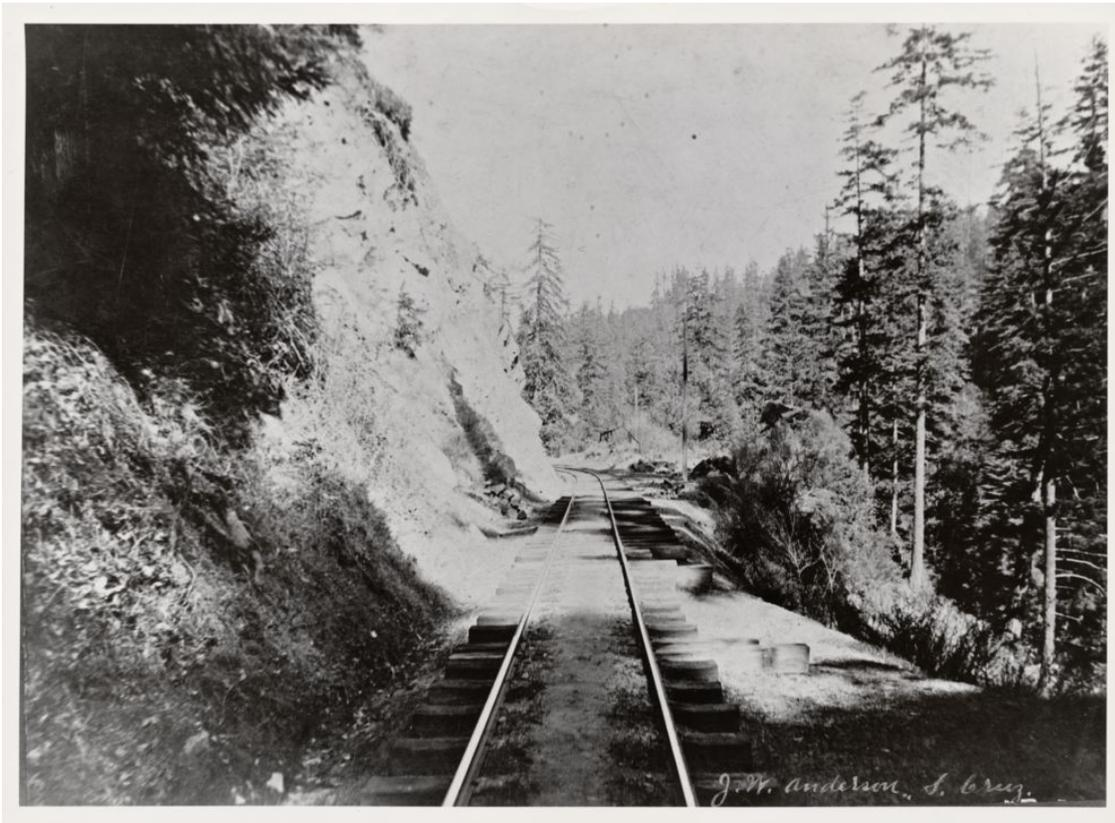
**Exhibit 2.** A photograph showing the expansion of either the Santa Cruz and Felton Railroad or the Felton and Pescadero railroad from narrow to broad-gauge in the proximity of Felton, c. 1905 (University of California, Santa Cruz Special Collections).
