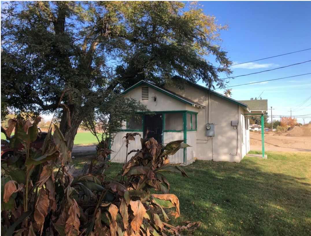
B) View of the south facing façade of the residence looking north. 11/29/20. Acc. #MM9271
