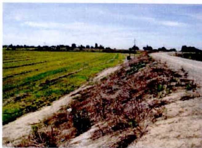
East site of levee – view to south
