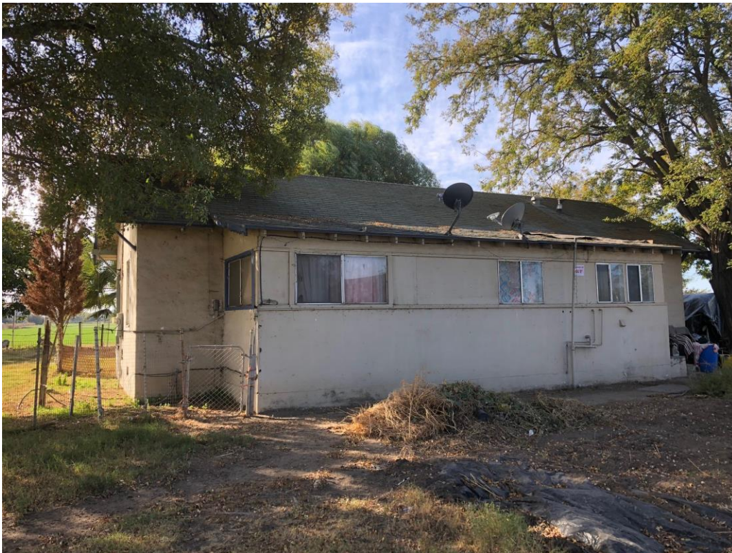
D) View of the north facing façade of the residence looking south. 11/29/20. Acc. #MM9269
