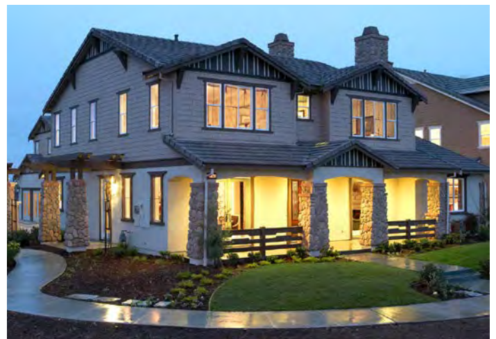
Wrapping porch around corner
