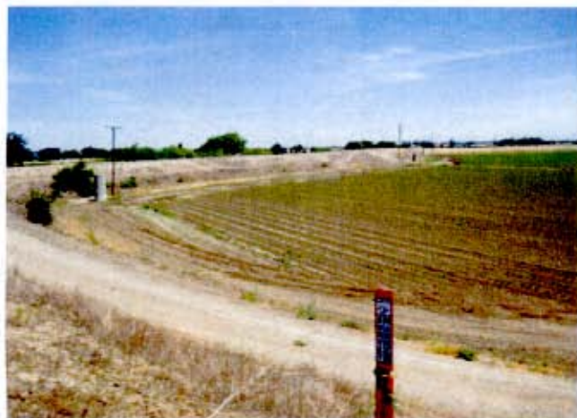
East side of levee and adjacent fields – view to north
