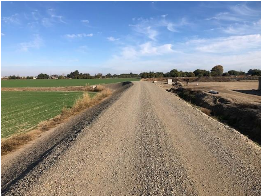
D) View of the terminus of the levee, project area to left, looking east. 11/23/20. Acc. #MM9308
