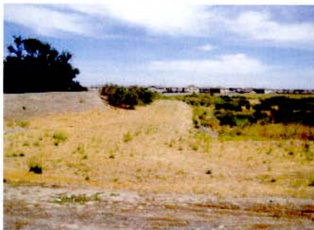
East side of levee and adjacent residential development – view to north
