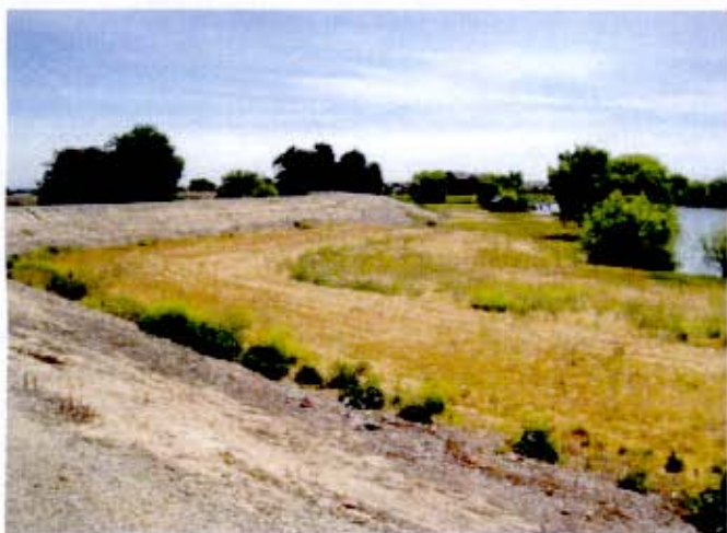
East site of levee – view to north.
