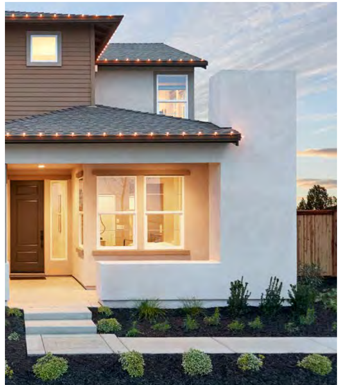
Smooth stucco application
