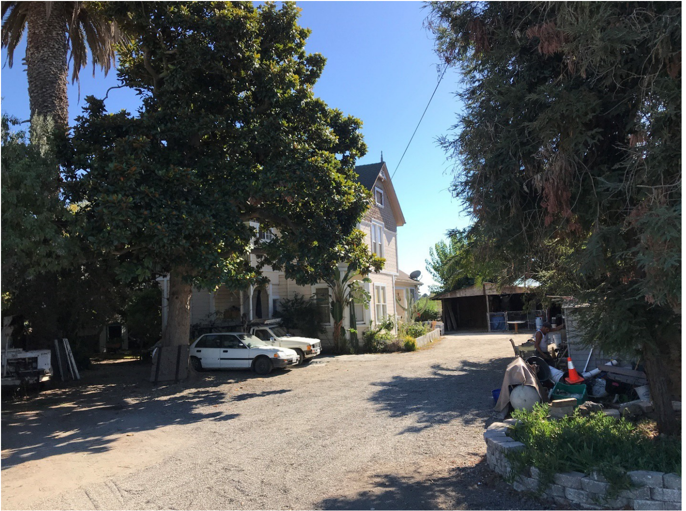
Photo 2. Facing south. Mature trees (Mulberry and Palm), farm house, and carport (right, rear).
