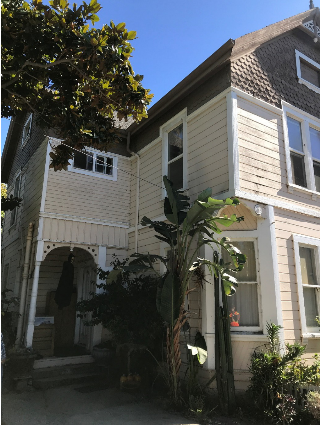
Photo 5. Facing southeast showing front entrance and second-story porch-to-bathroom conversion.
