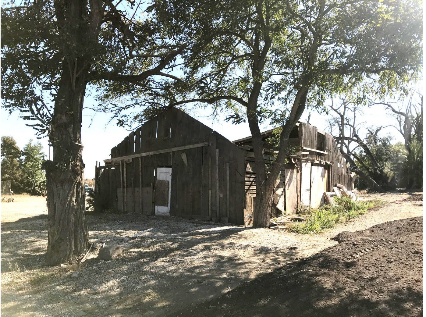
Photo 7. Facing southeast toward the reconstructed barn, a non-contributing feature.
