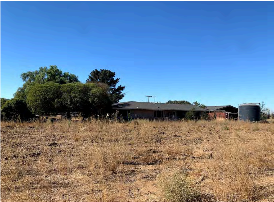
Photo 4: View of the existing vacant residence on the project site.
