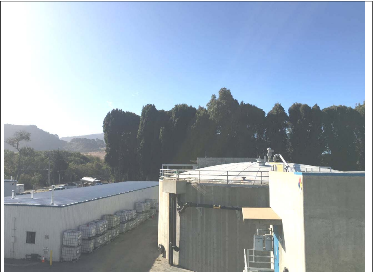
Photo 1: Taken from on top of an existing building inside the WWTP looking Southeasterly at southern property line.
