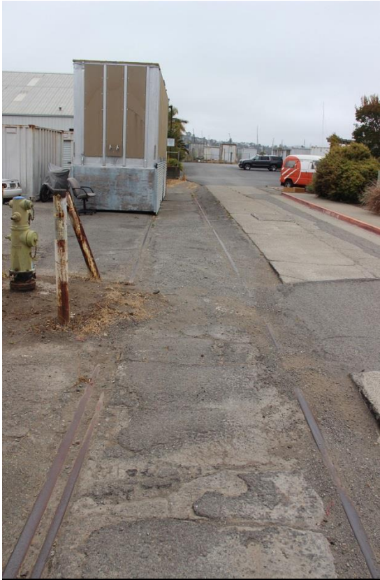
Figure 4. Track segment, looking northeast.
