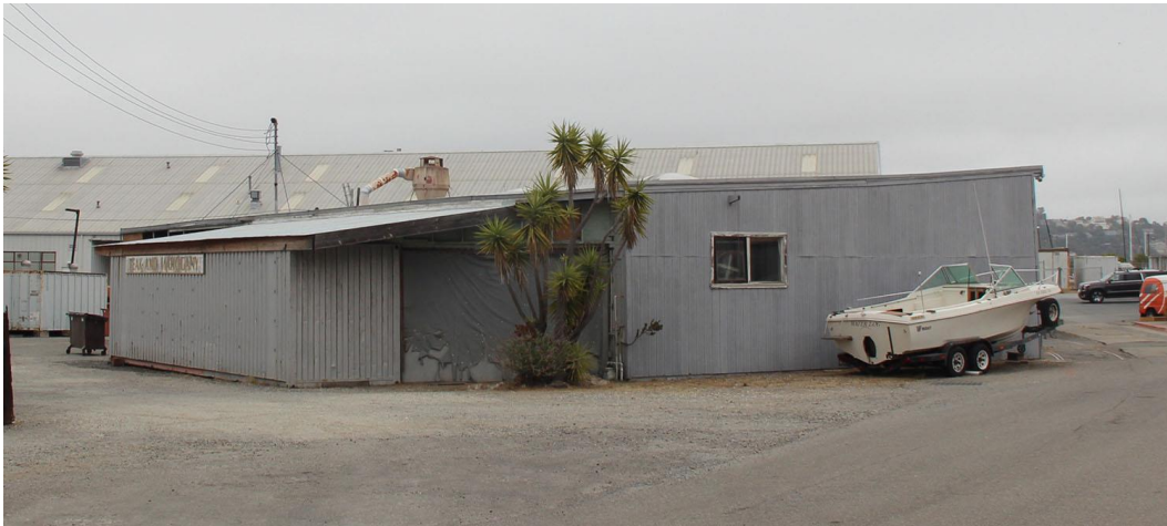
Figure 3. Building 13 Annex at 60D Liberty Ship Way.
