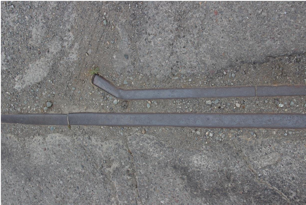
Figure 6. Detail of track segment showing twin rails on north side.
