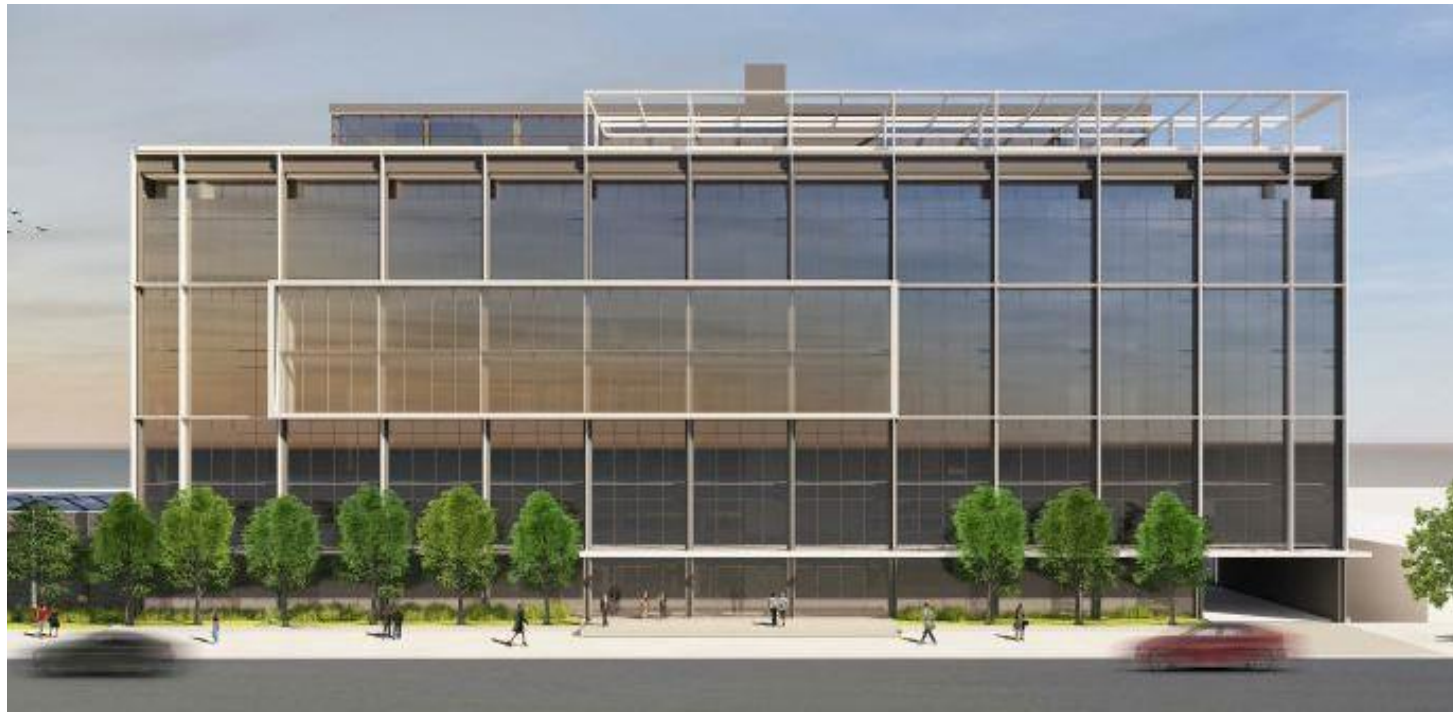
Forward facing view of Building A frontage along Pacific Coast Highway/Highway 1/Sepulveda Boulevard showing the proposed improvements.
