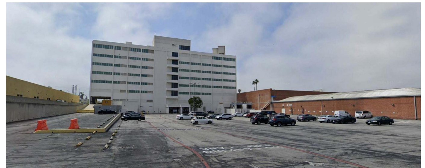
View facing west from the future Building C location showing the east sides of Building A and Building B.
