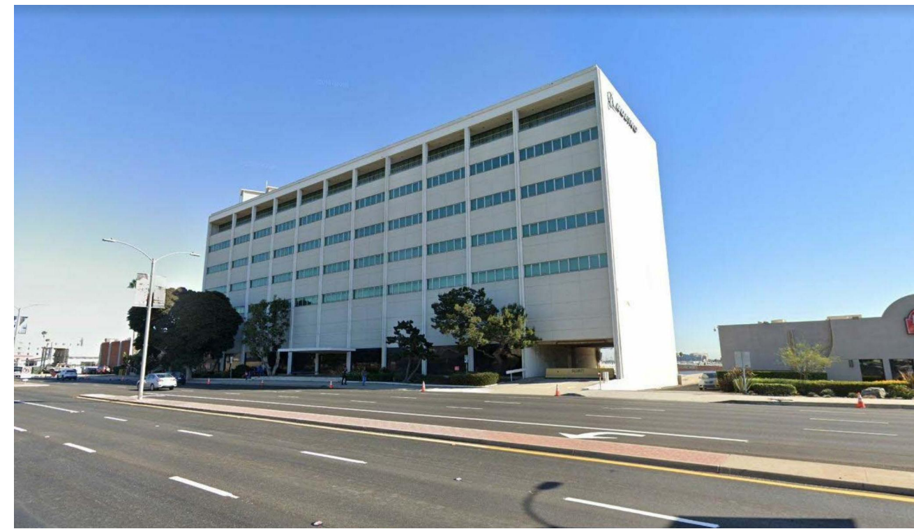
View facing northeast, showing Building A frontage along PCH.
