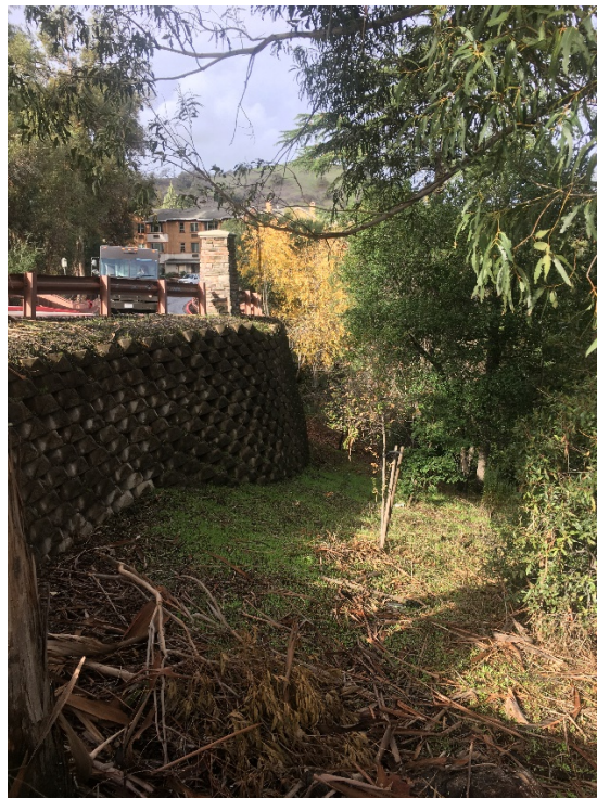
West side of bridge/retaining wall structure
