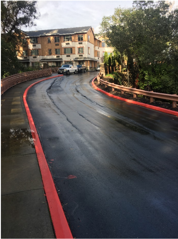
Driveway to facility
