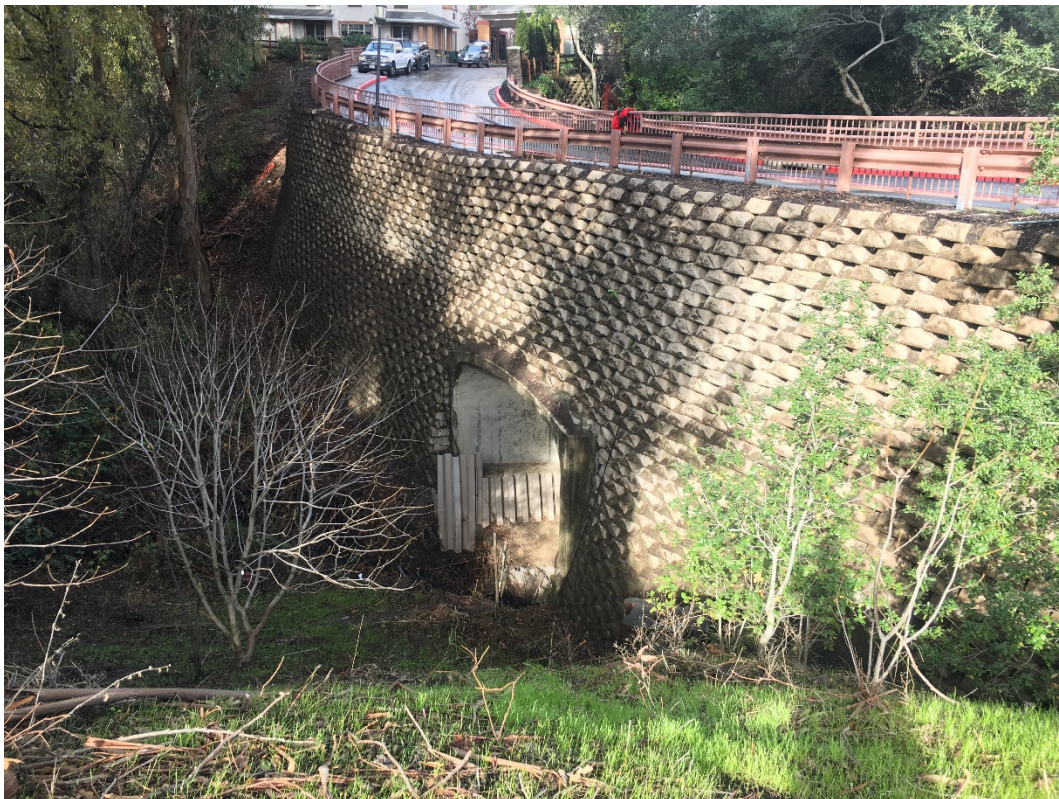
East side of bridge/retaining wall structure, viewed from Pleasant Hill Road
