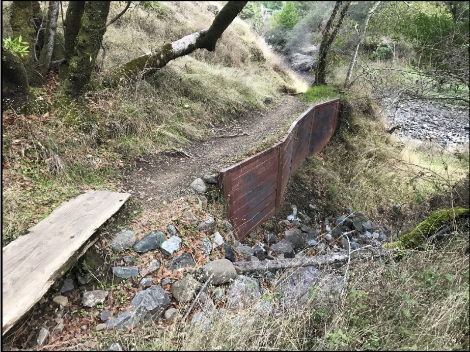
Photo 8: Existing Puncheon and Retaining Wall on the High Water Trail
