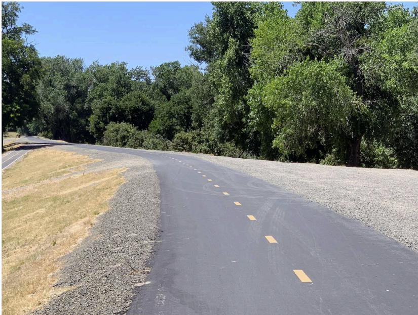
View of similarly proposed Levee Top trail alignment from Phase I of the Two Rivers Trail near Township 9 Park, facing west.
