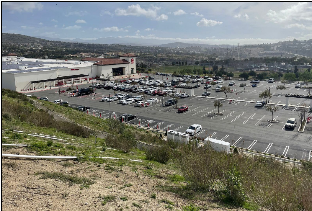
PHOTOGRAPH 2 Site B Looking Southeast
