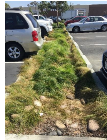
Swale with trees between parking
