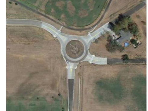
Aerial view of constructed roundabout with permeable pavement and biofiltration with connection to storm drain
