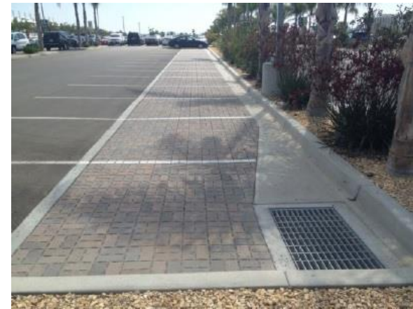
Green parking lot with permeable pavement in parking stall
