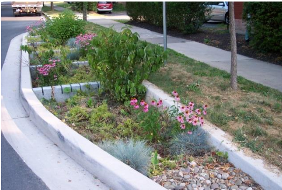
Curb extension with planter box
