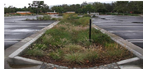
Swale in Island
