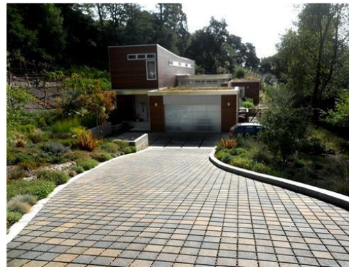
Permeable pavement driveway
