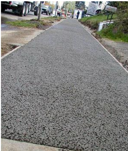
Pervious concrete sidewalk
