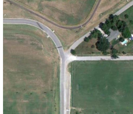
Aerial view of rural intersection before roundabout
