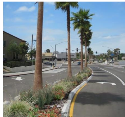
Green street depressed median with curb cuts and planter/swale
