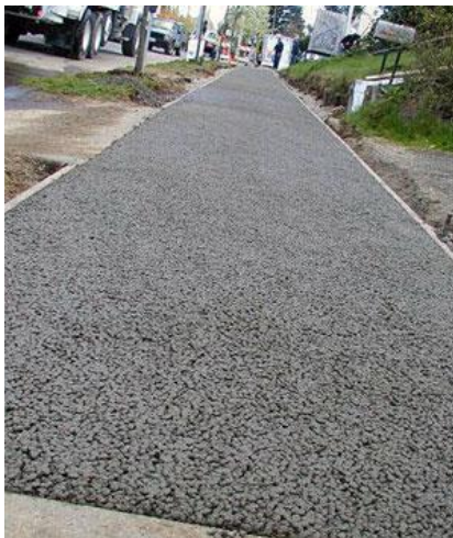
Pervious concrete sidewalk
