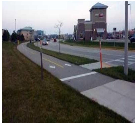
Porous asphalt pathway
