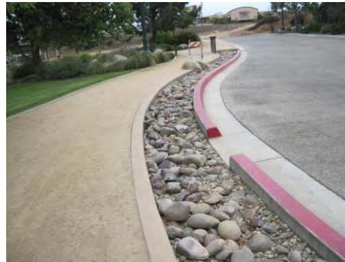
DG pathway with rock swale
