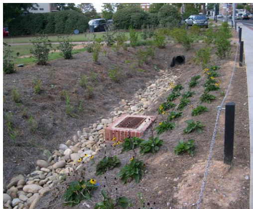
Swale outside of parking lot
