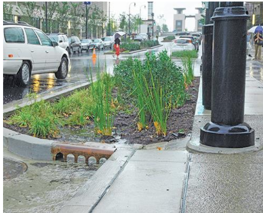
Curb extension with planter box
