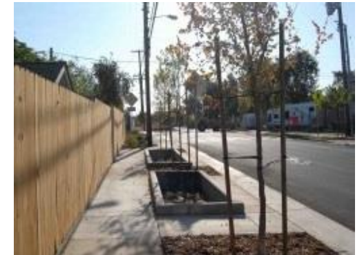
Reconstructed Road with Trees and planter boxes
