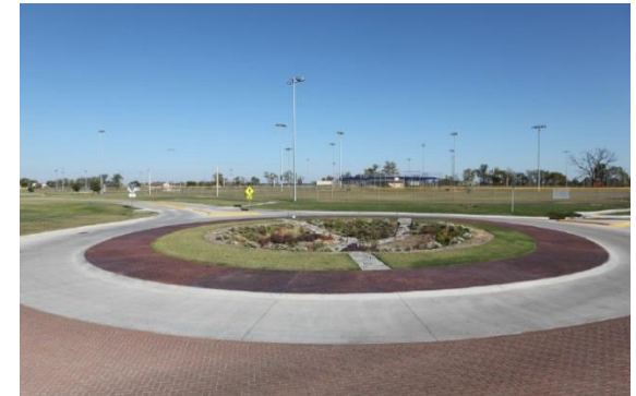
Street view of same roundabout
