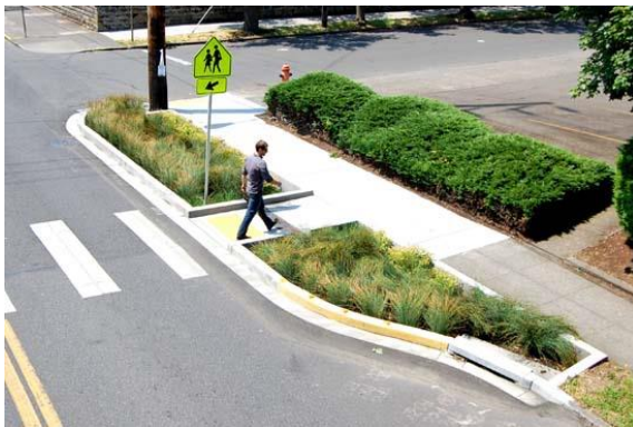
Bulb-out planter box at intersection
