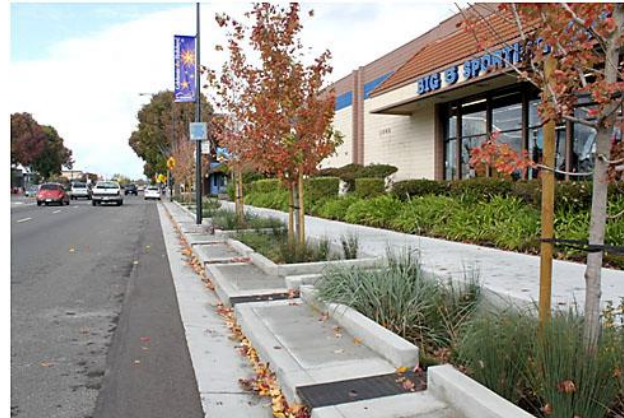
Road retrofit with planter boxes and trees
