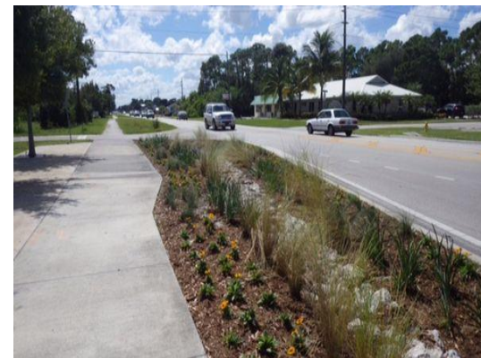
Swale adjacent to road
