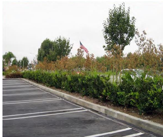
Conventional parking lot with Asphalt Concrete in stall
