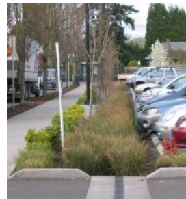
Bioswale adjacent to parking and sidewalk
