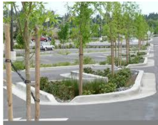
Biofiltration with trees in Island
