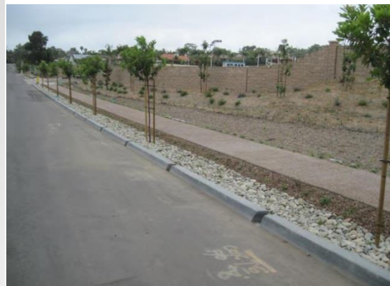
Rock swale adjacent to road
