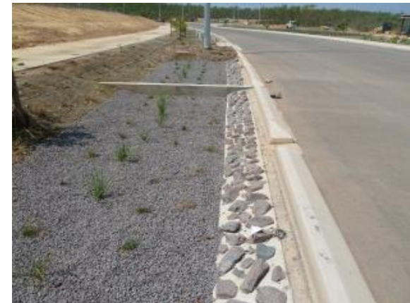
Rock swale adjacent to road
