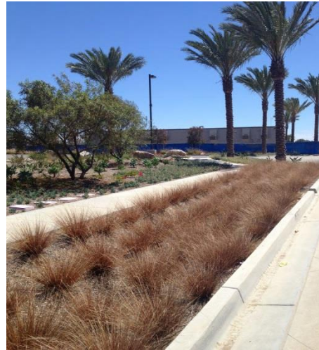
Swale adjacent to road
