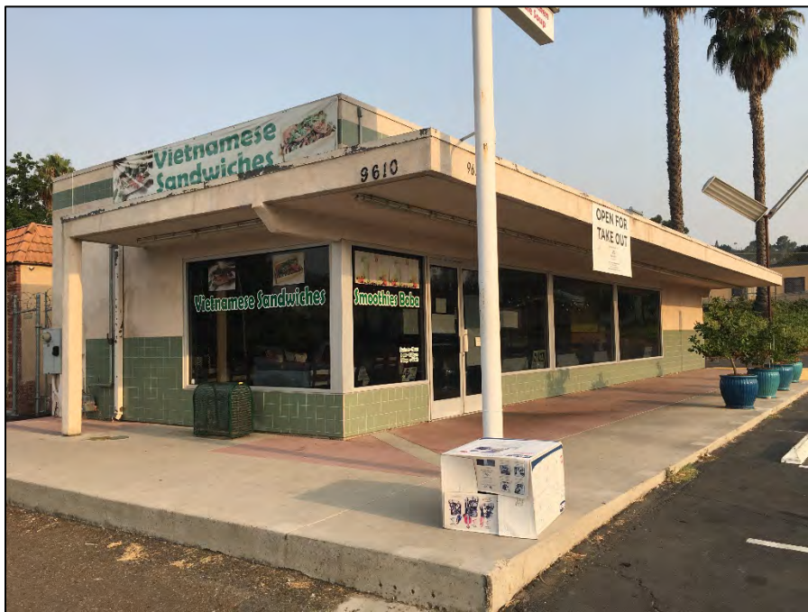
Figure 2. P-37-039110; Commercial building, southeastern façade (view northwest; September 9, 2020).
