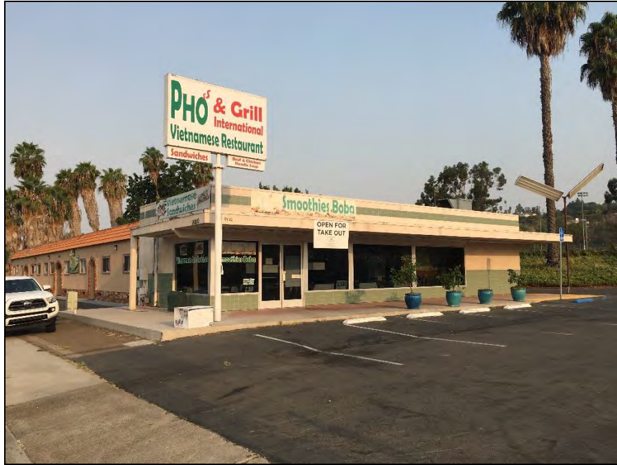
CDO-01; Commercial building, southeastern facade (view northwest; September 9, 2020).
