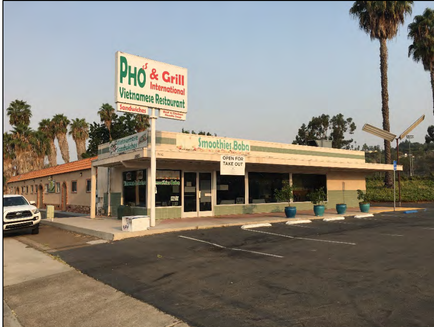
Figure 3. P-37-039110; Commercial building, southeastern façade (view northwest; September 9, 2020).
