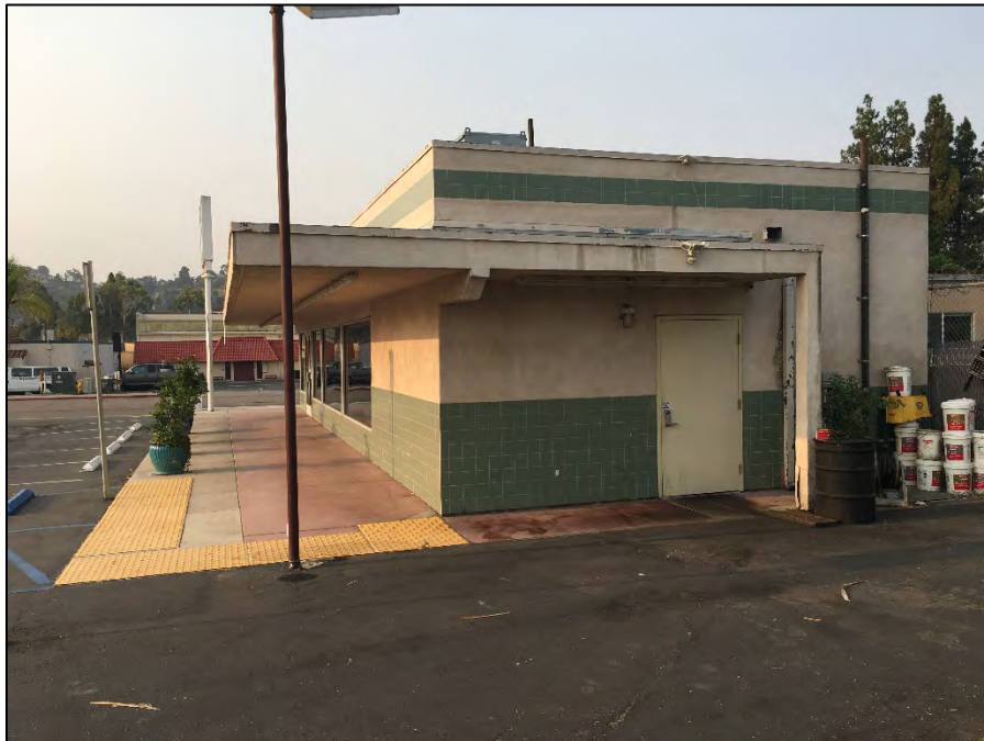
Figure 4. P-37-039110; Commercial building, northern façade (view south; September 9, 2020).
