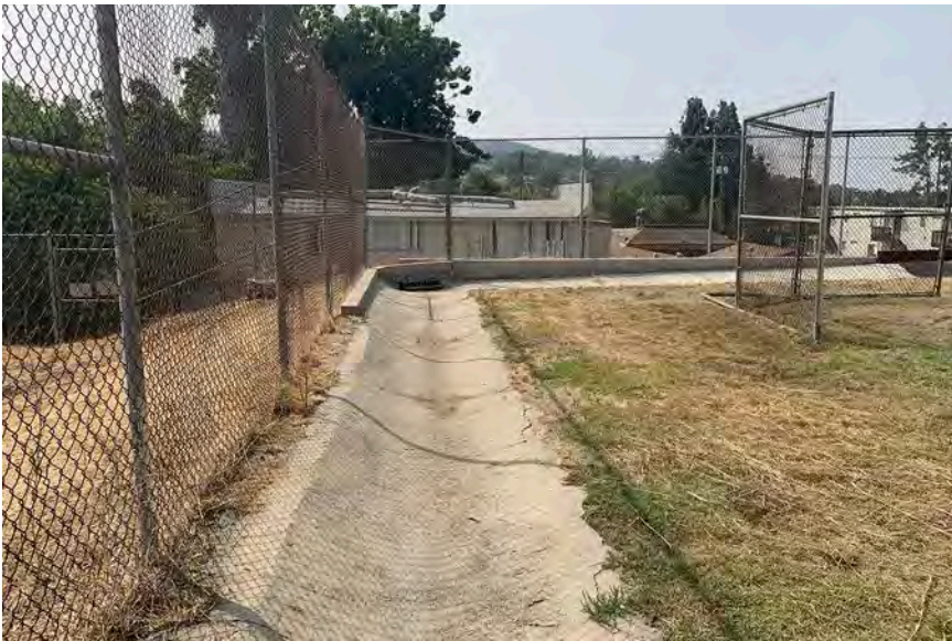
View of culvert in southwestern portion of the subject site.
