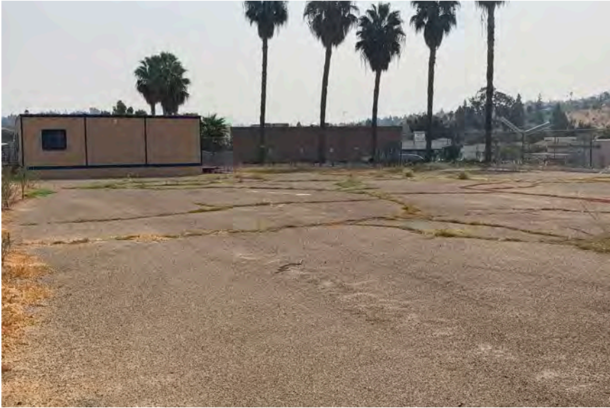
View of paved surface in southern portion of the subject site.
