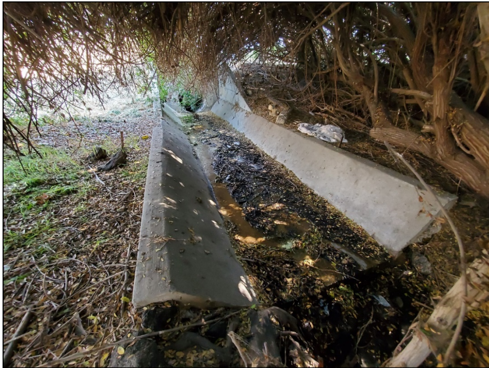
Photo 6: View of the storm drain outlet, facing north.
