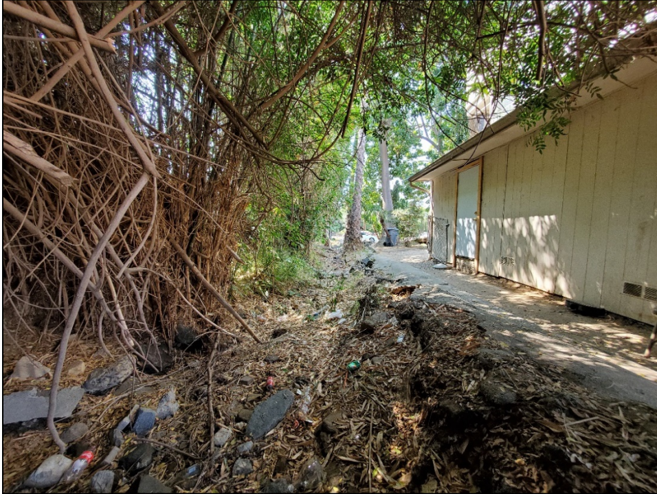
Photo 8: View of the storm water drainage, facing south.
