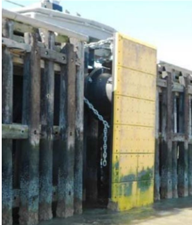
Figure 2.10 – Typical Super Cone Fender
