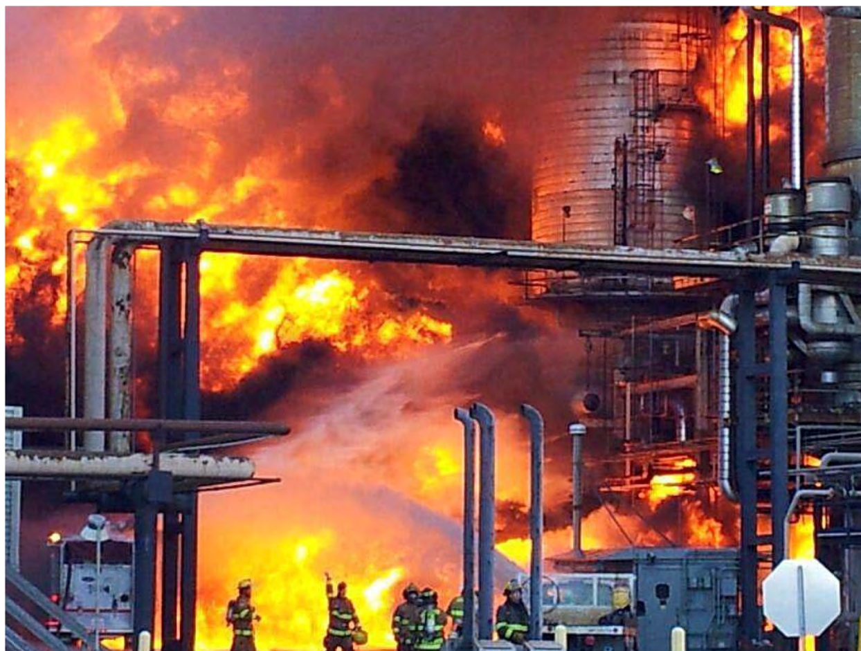
Chevron Richmond Refinery, 6 Aug 2012. Image: CSB
