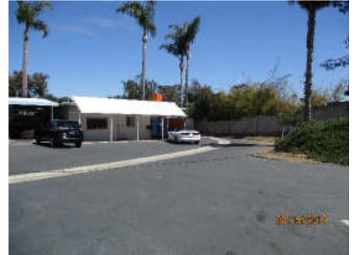
South side of property facing east
