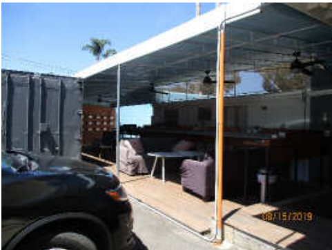
Backside of office building facing northeast
