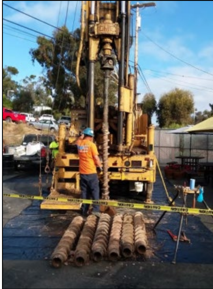
Figure 3-2. Drilling Operations, September 17, 2019
