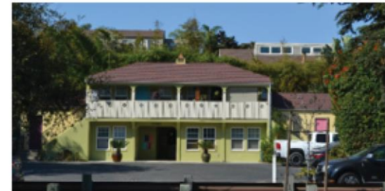
Photo 12: Existing commercial use located south of project site (west side of Highway 101).
