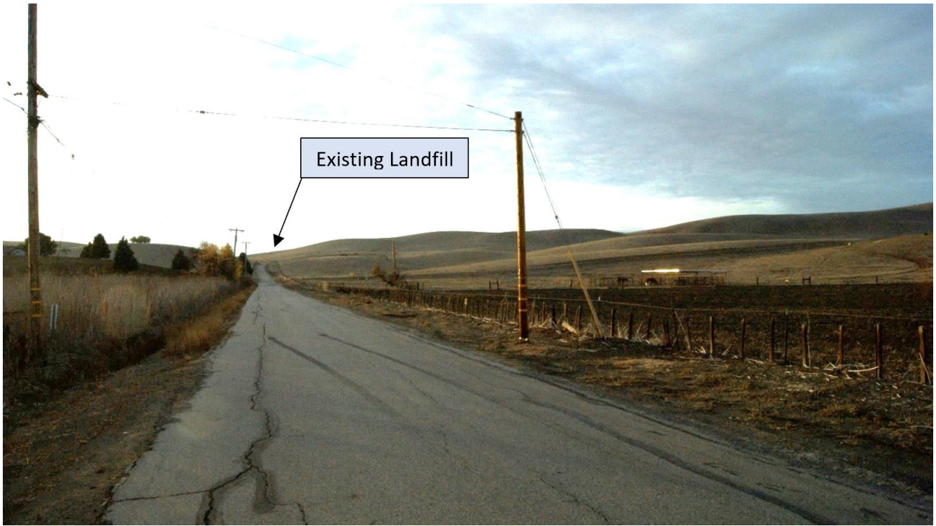
View facing west on John Smith Road toward the existing landfill
