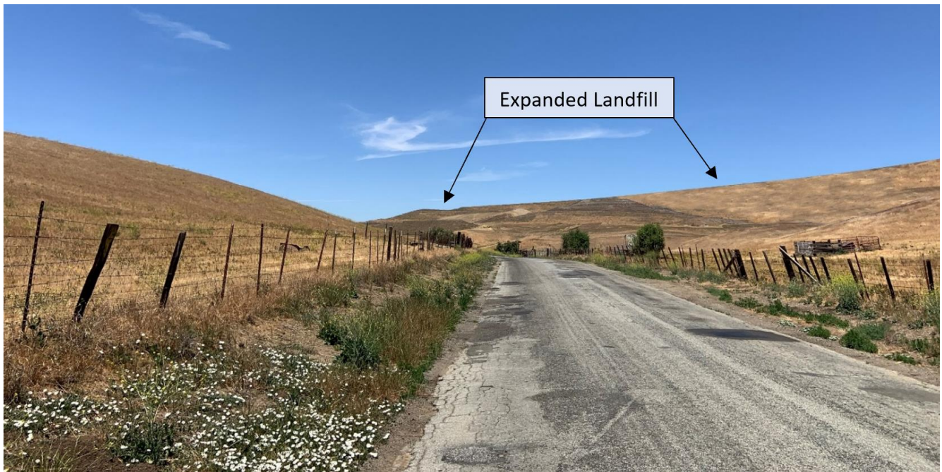
Simulated view facing west on John Smith Road toward the proposed project at full buildout. The change in elevation with the proposed project is visible at the horizon directly above and to the right of the roadway. Native grasses have been added to the filled landfill slopes.
