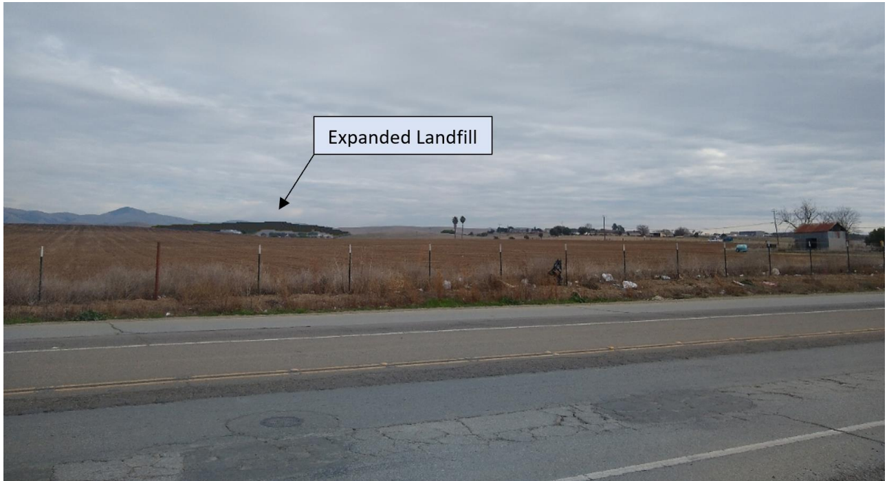
Simulated view from Fairview Road looking east (just north of John Smith Road) toward the proposed project at full buildout. The proposed project is visible at left in the middleground.
