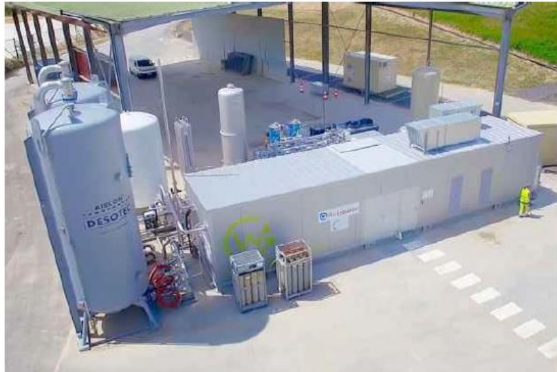
BIOGAS: 45-50% CH 4 ; 0-3% O 2 ; 7,000 ppmv H 2 S ; 5-20% N 2 200,000 TONS OF WASTE PER YEAR
