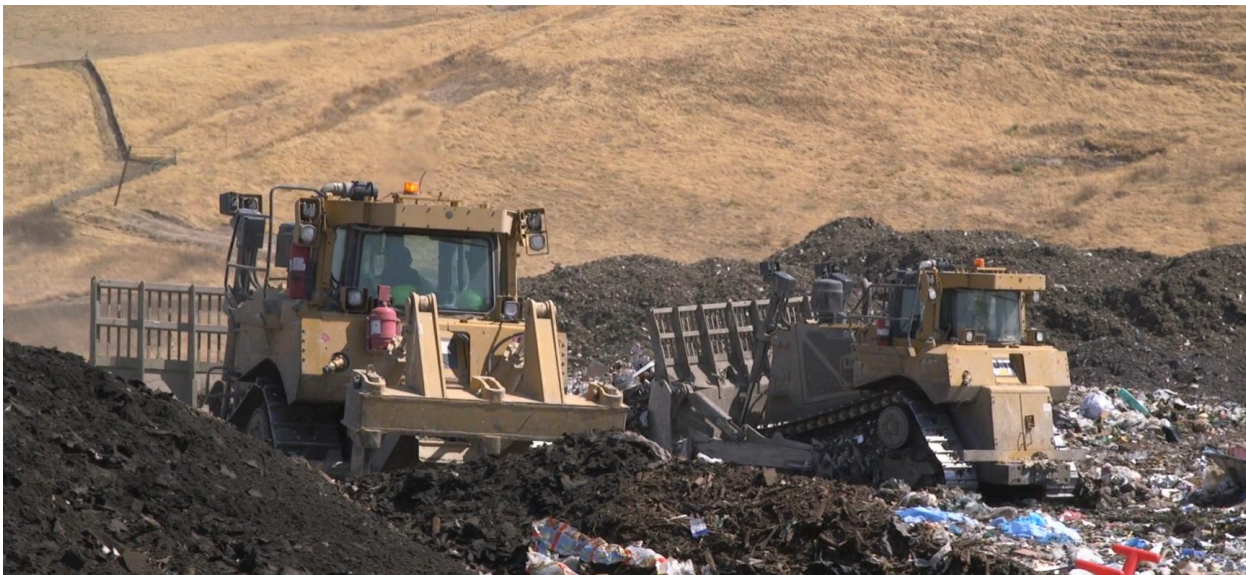
Typical Waste Compacting at a Landfill Working Face
