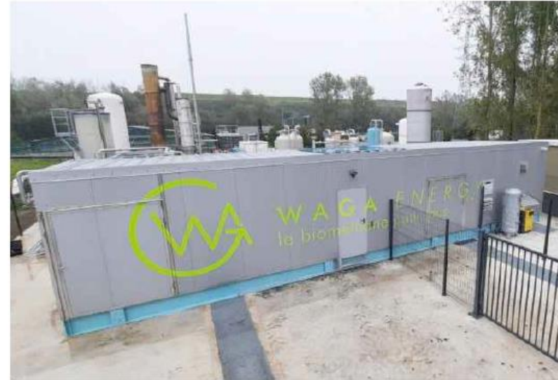
BIOGAS: 40-50% CH 4 ; 0-3% O 2 ; 300 ppmv H 2 S ; 5-20% N 2 600,000 TONS OF WASTE PER YEAR
