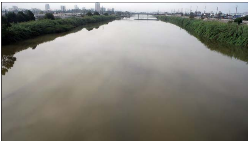
View from Pacific Coast Highway of the Los Angeles River Channel Reach No. 114.
