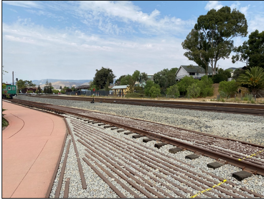
Photograph 1. North end of BSA, view looking north toward existing Pacific Surfliner Layover Facility
